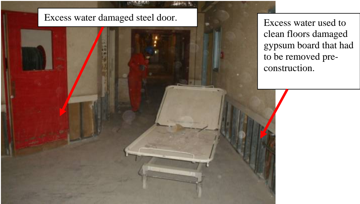
Site Photo 5. Hallway prior to renovation. (USACE photo taken 18 June 2005)
