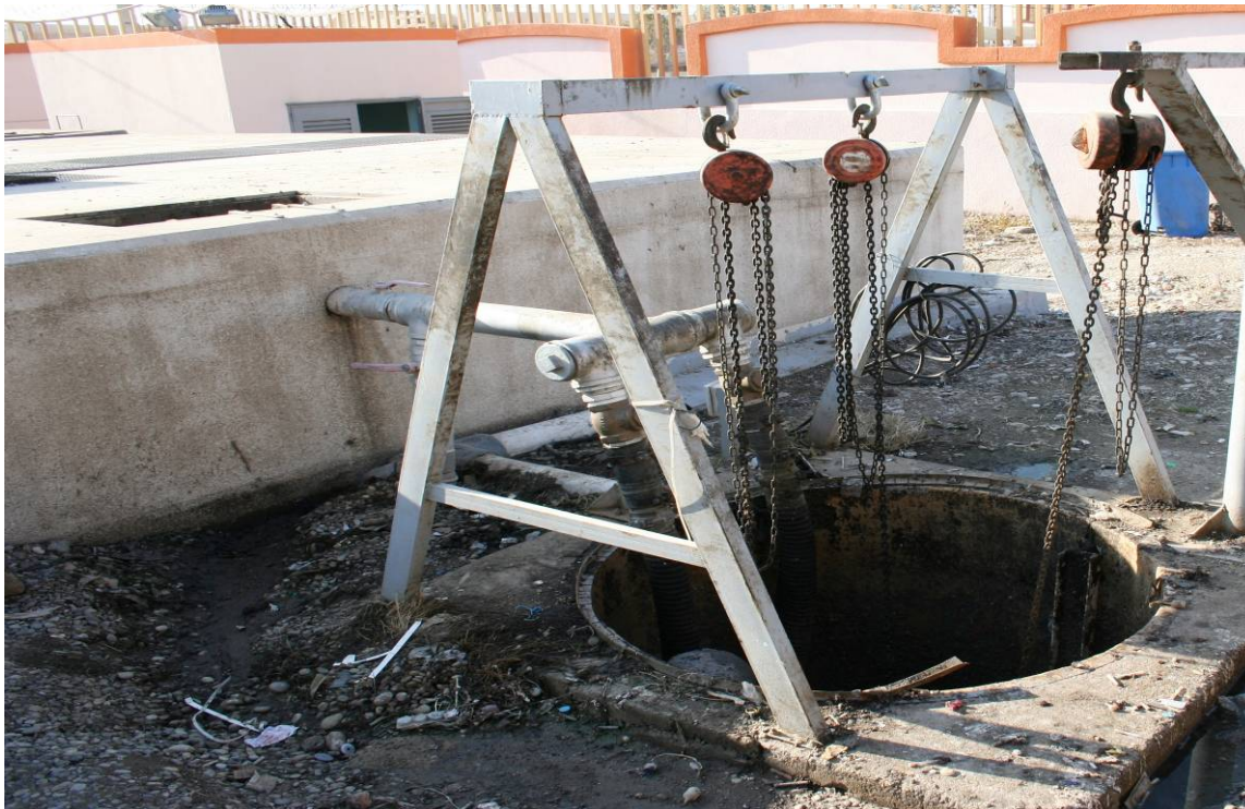
Site Photo 18. During the inspection, the area between the cesspool and septic tank was littered with ineffectively burned medical waste materials.
