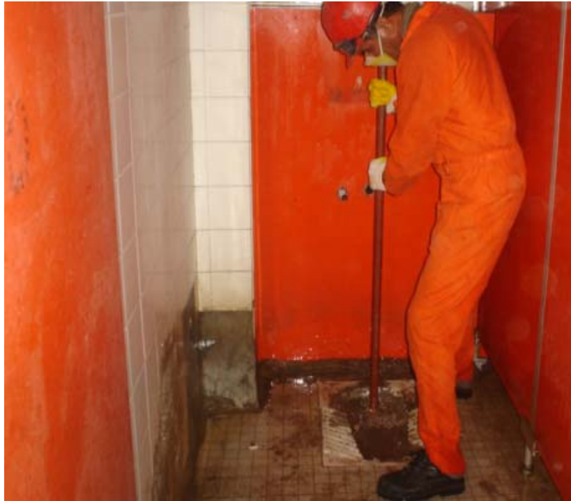
Site Photo 3. Water closet/toilet prior to renovation. (USACE photo taken 11 August 2005)
