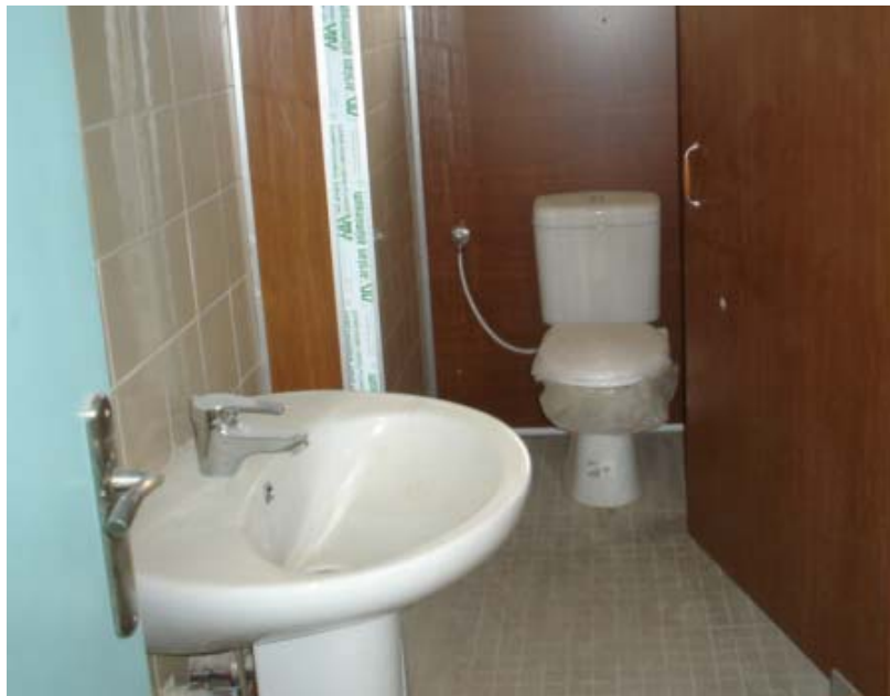
Site Photo 4. Toilet with sink following renovation. (USACE photo taken 8 Jan 2006)
