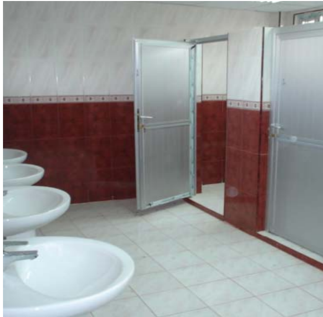
Site Photo 2. External toilet following renovation. (USACE photo taken 18 Jan 2006)
