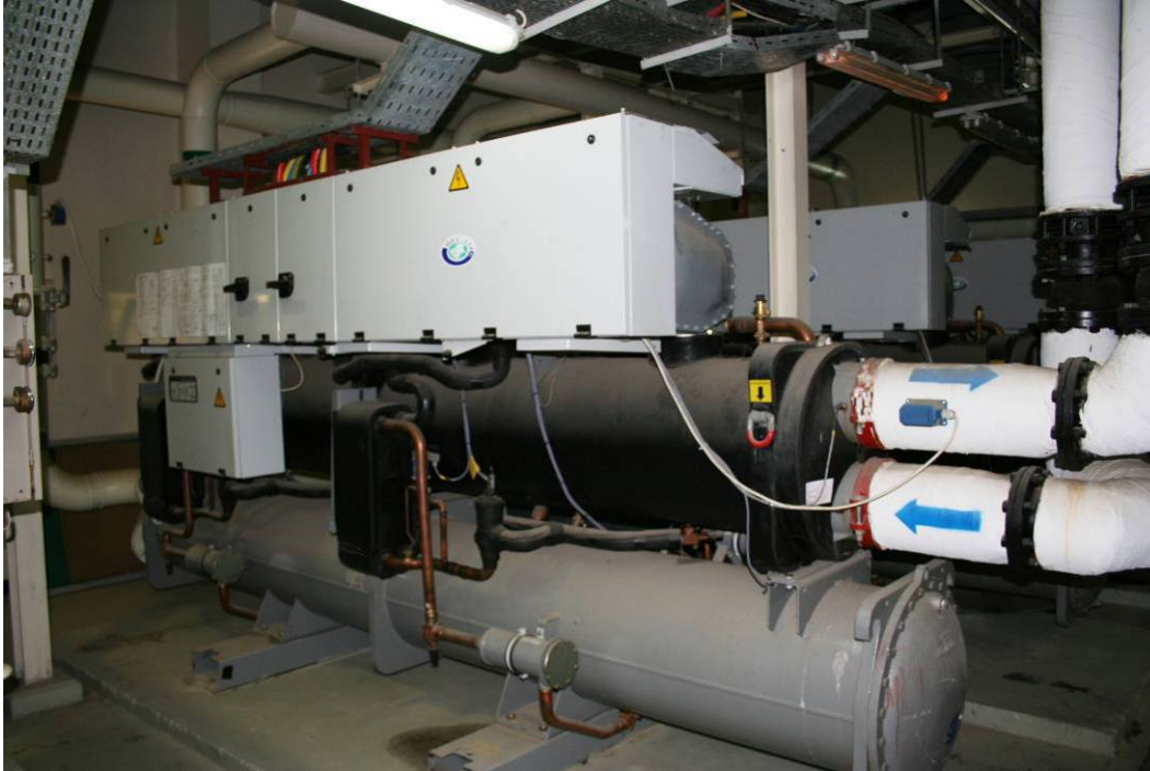
Site Photo 29. Chiller installation appeared satisfactory.
