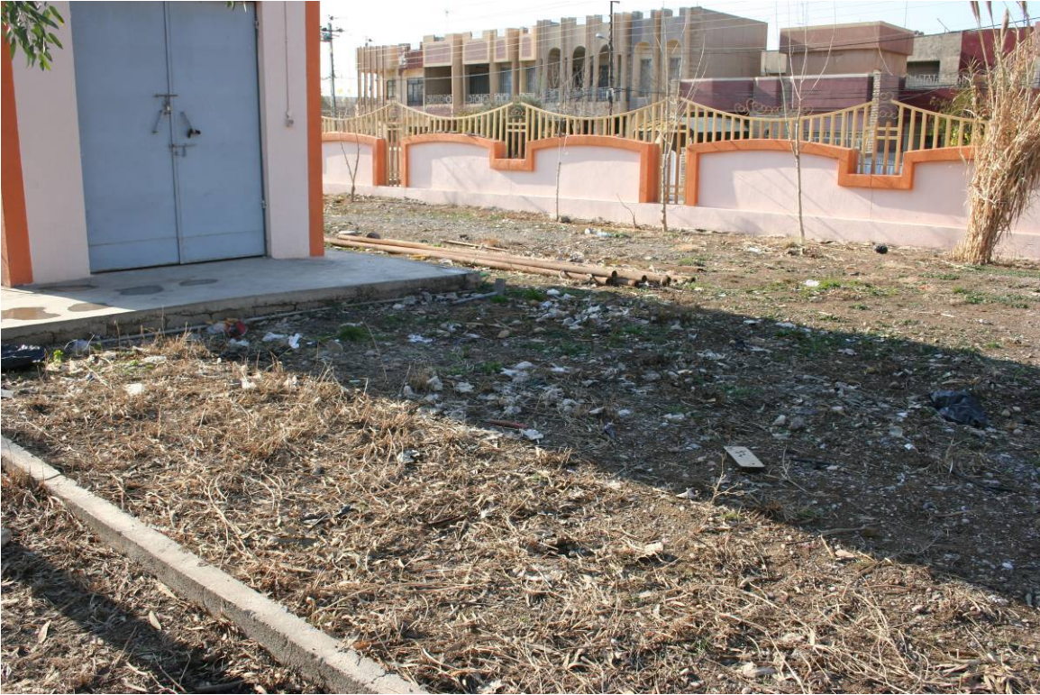
Site Photo 12. Medical waste materials scattered on the ground area in front of the new incinerator.
