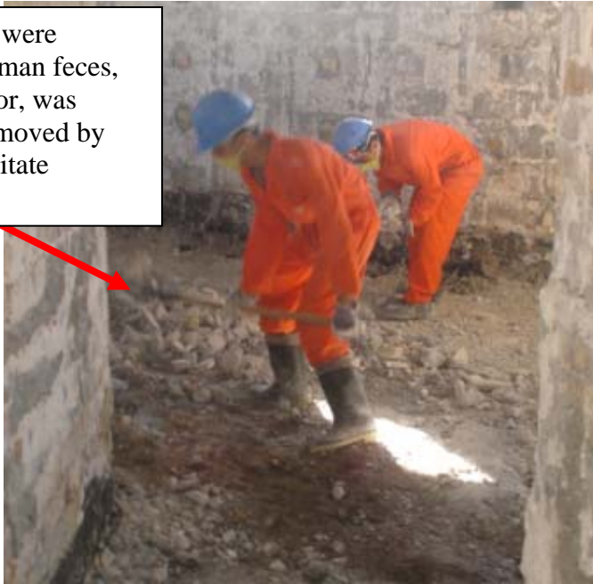
Site Photo 1. External toilet prior to renovation. (USACE photo taken 18 June 2006)
