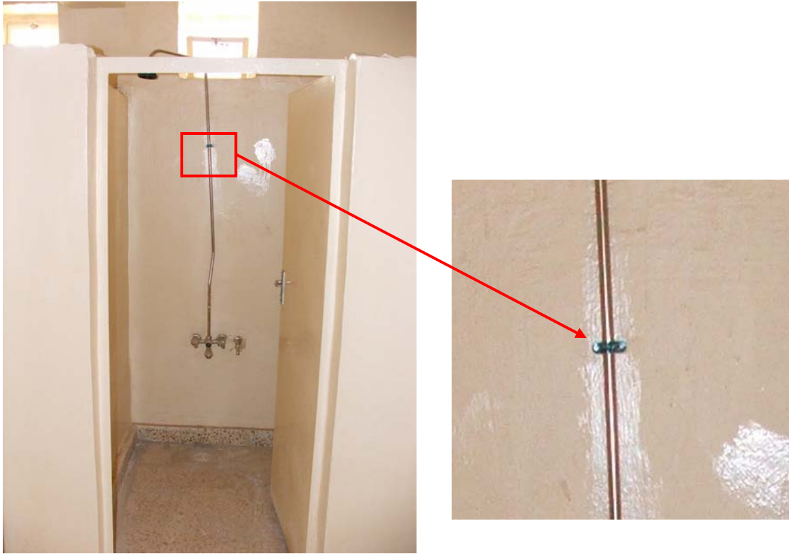
Site Photos 26 and 27. Single screw clamp holding the thin metal water pipe to the wall.
