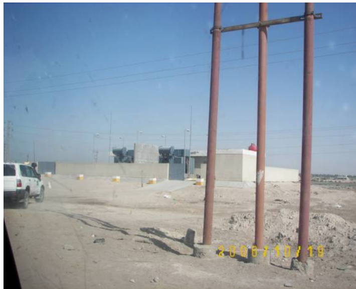
Site Photo 2. Al Hamdan substation perimeter walls
