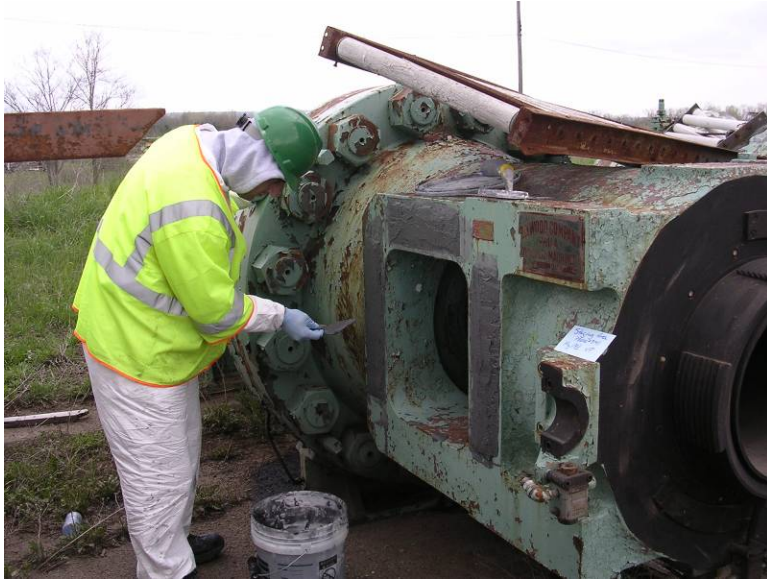
Figure 5-28. BTS paste being applied to press 14.
