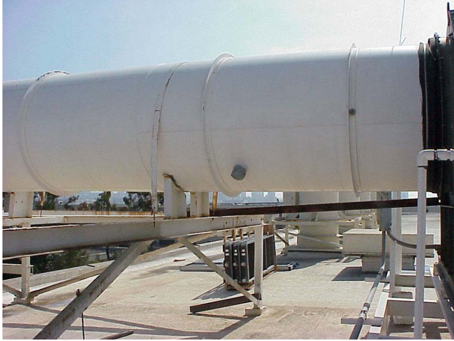
Figure 2-2. Sampling port on chromium plating bath exhaust on roof of building at NADEP.
