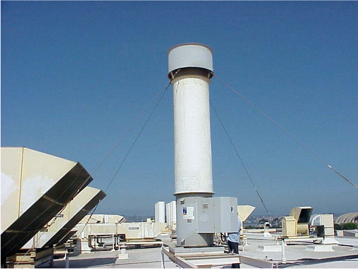
Figure 2-3. Electroless nickel plating bath exhaust stack on roof of building at NADEP.
