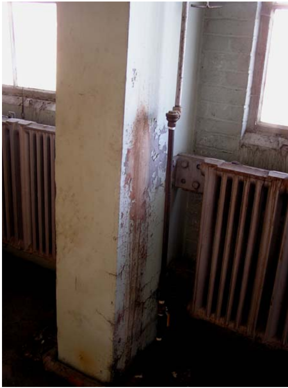
Figure 27: Pedestal 5 north: largely intact, with diagonal crack at 50".
