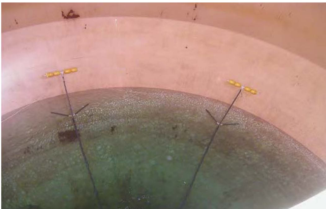
Figure 15. Top view of anode supports as tank fills with water.
