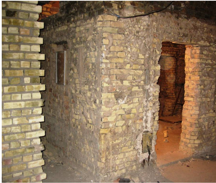
Site Photo 7. Existing brick walls in building B1 after demolition of interior finishes
