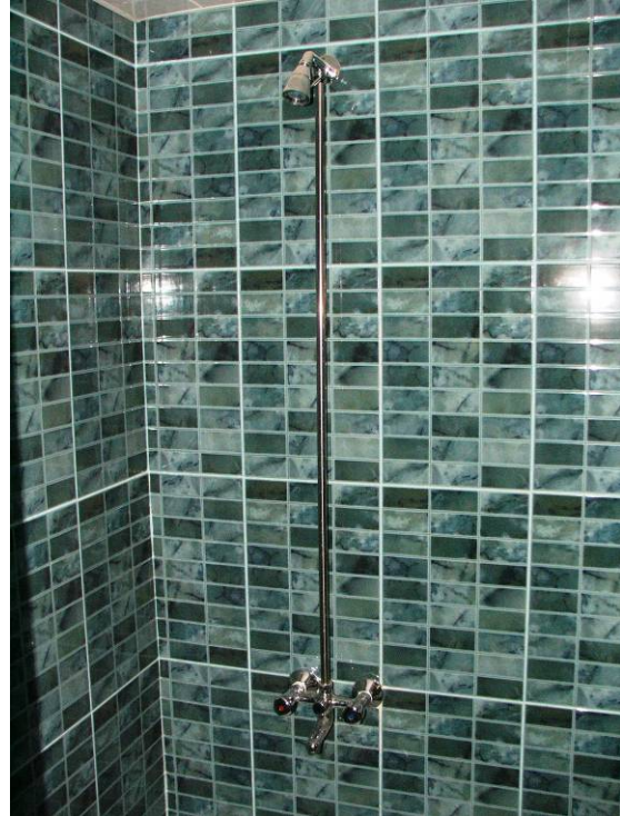
Site Photo 3. Renovated patient bathroom shower assembly
