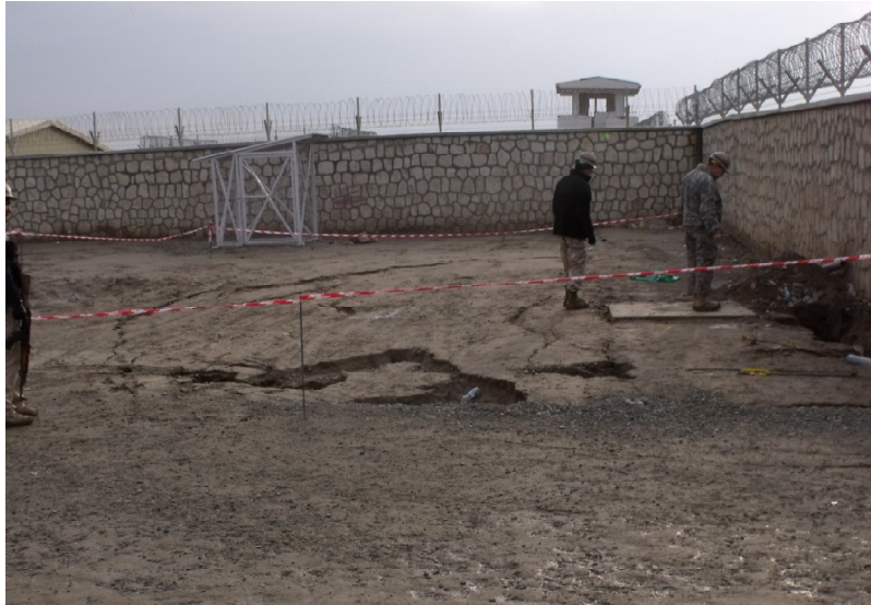
Photo 5: Settling along the Embedded Training Team Compound Wall at Kunduz ANA Garrison
