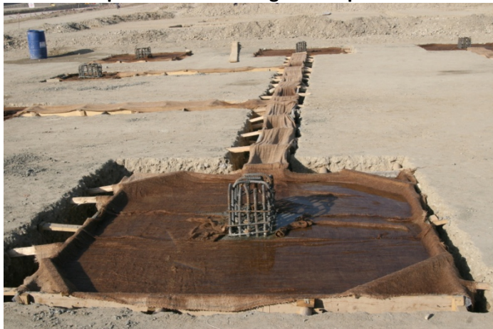
Photo 1: Proper Concrete Curing Techniques at the Gamberi ANA Garrison
