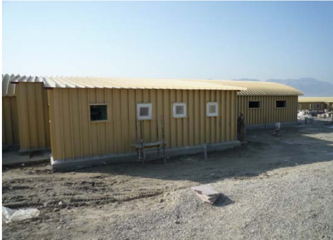
Photo 2: K-span Building Properly Installed at the Gamberi ANA Garrison
