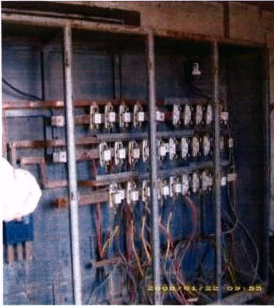
Photo 2 and 3: Power Plant 1 PRE-IMPROVEMENT —The main power distribution panels at Power Plant 1 as they appeared prior to the renovation work done in the spring 2008; showing no cover doors and high voltage wires lying exposed on the ground instead of being run through power cable canals that lead to the generators. (Photo courtesy of Khowst PRT)
