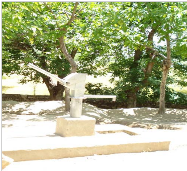
Site Photo 4: During the onsite visit to the school, SIGAR inspectors found that the water pump installed 3 months earlier was not operable. (Photo provided by SIGAR)
