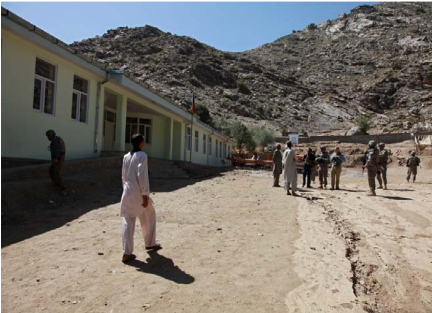
Site Photo 7: View of school grounds less than one month after grading work was completed showing signs of site erosion. (Photo provided by Kapisa PRT)
