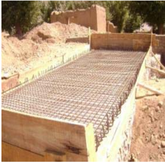
Site Photo 8: A rebar and wood formwork prepared to construct one of the 26 slab culverts required by the design plan. (Photo provided by Kapisa PRT)
