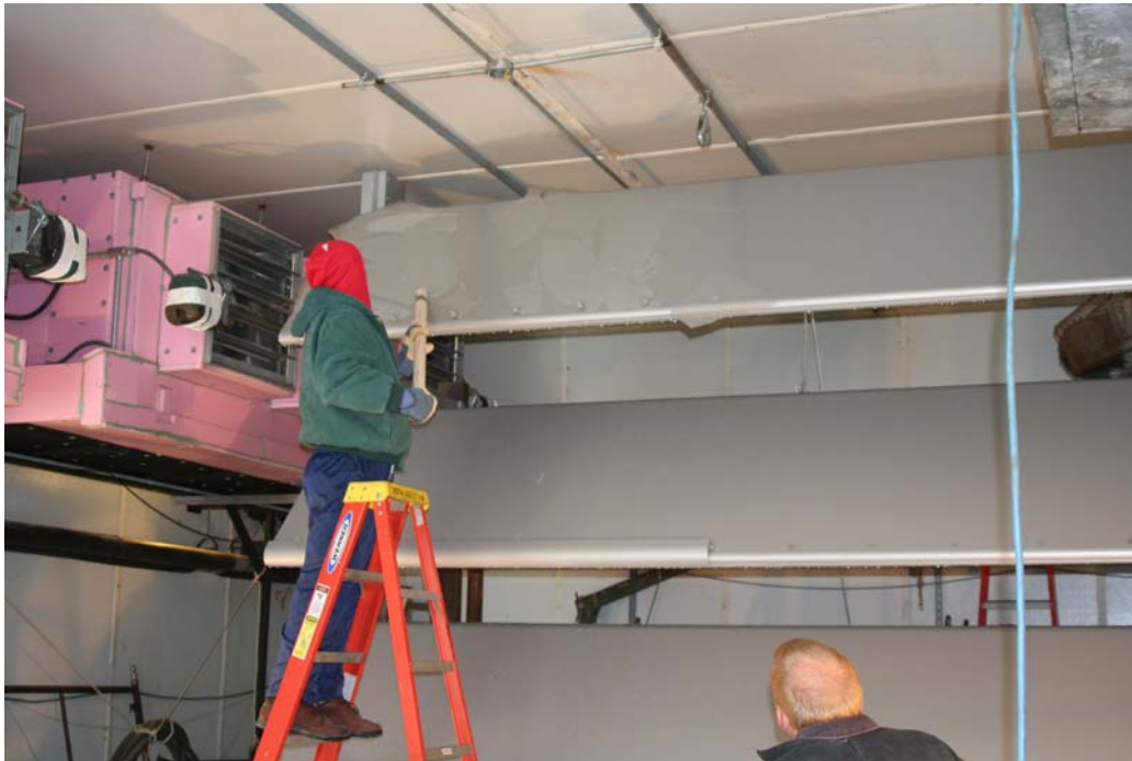
Figure 1.14. Manually removing the ice above the IRD on fin A4 is a very labor-intensive process.
