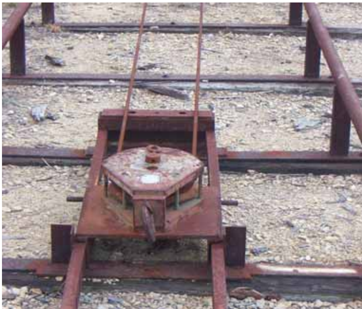
Figure 492. Cable pulley system on moving target track, Fort Bragg, NC, 17 May 2006.
