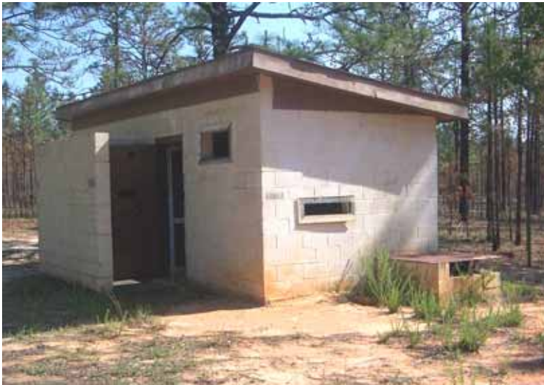
Figure 543. Range latrine, Fort Bragg, NC, 17 May 2006.
