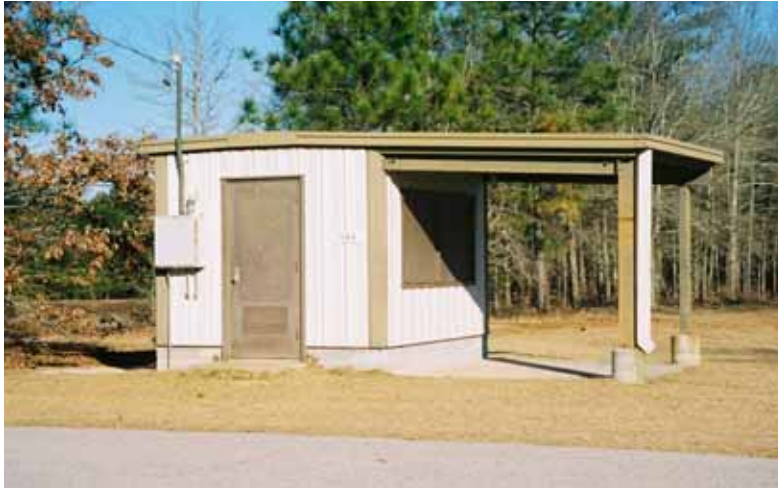
Figure 535. 1987 Building 485 range storage, Fort Gordon, January 2004.
