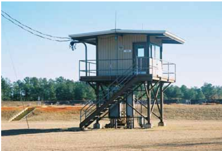
Figure 517. 1987 Range Bldg 486, Fort Gordon, GA, January 2004.
