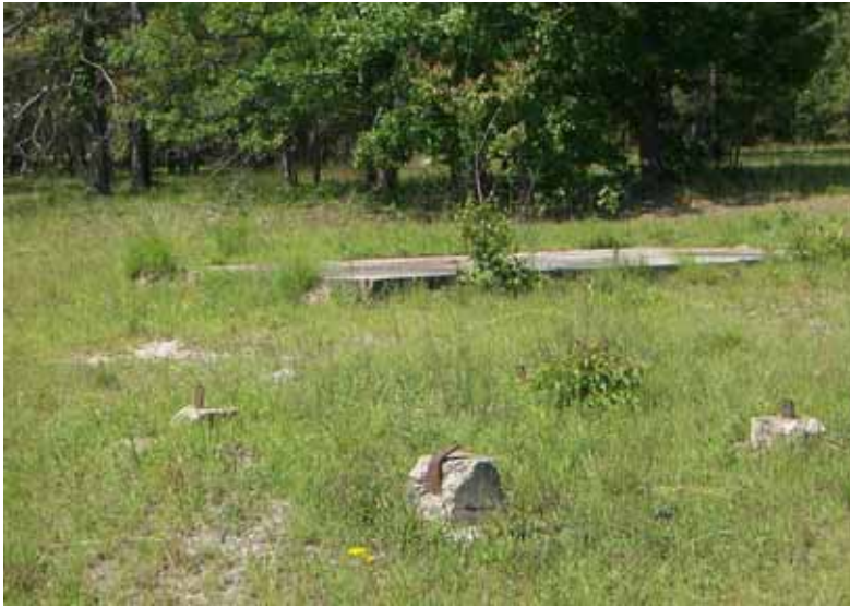
Figure 524. Abandoned known distance range (foundations of observation tower and range building), Fort Bragg, NC, 17 May 2006.
