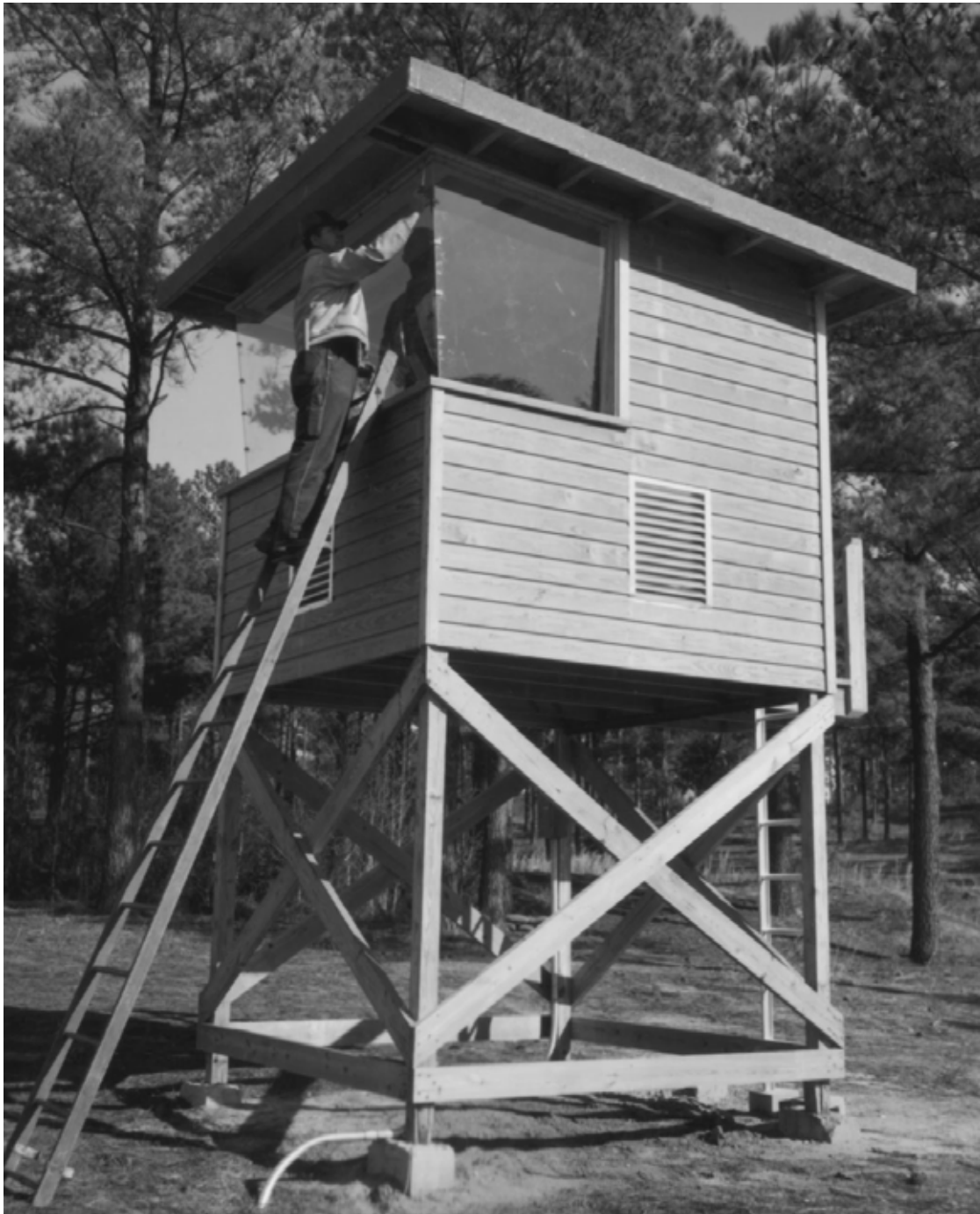
Figure 108. New rifle range control tower that is an essential component of the rifle ranges at Fort Jackson, SC, 14 January 1964 (NARA College Park, RG 111-SC post-1955, box 384, photo SC607734).
