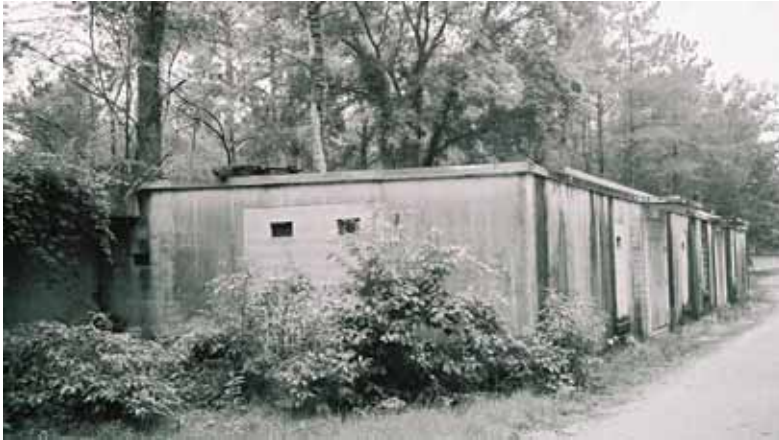
Figure 527. Remains of WWII known distance range target butt, latrine, and target storage, Fort Jackson, SC (SCARNG), June 2004.
