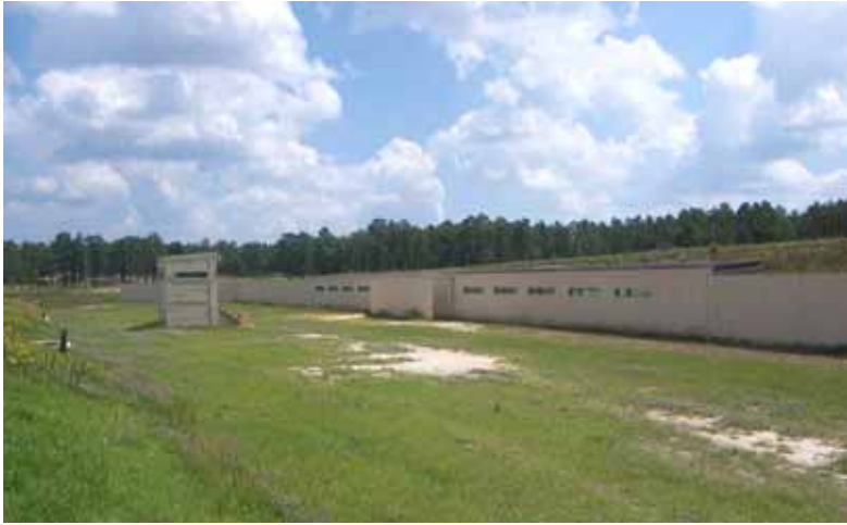
Figure 499. Grenade range protection walls, Fort Bragg, NC, 17 May 2006.
