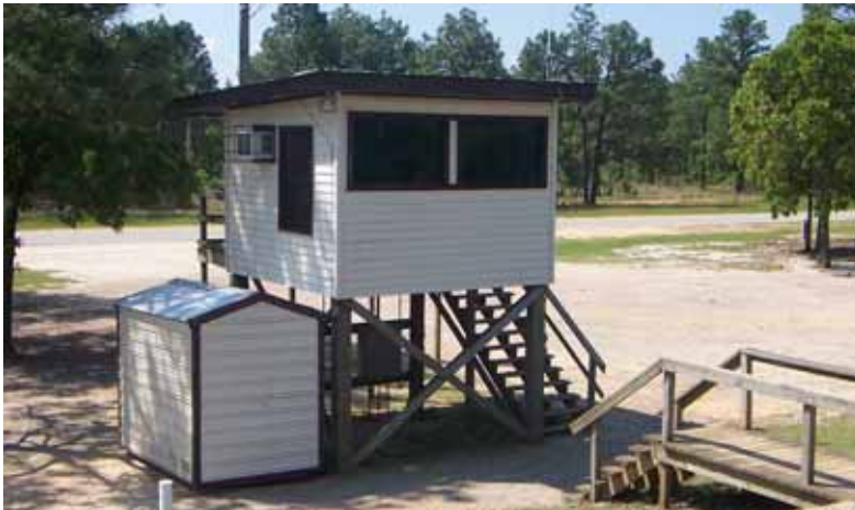
Figure 522. Observation tower, Fort Bragg, NC, 17 May 2006.
