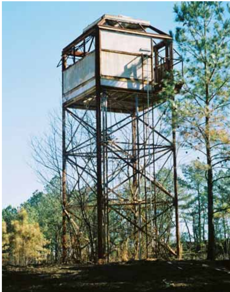
Figure 515. 1966 Observation tower near Old Range #19, Fort Gordon, GA, January 2004.
