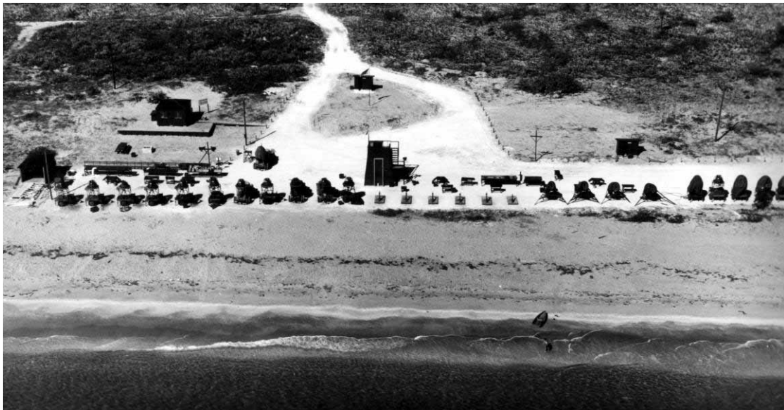
Figure 243. Beach firing range at NAS Fort Lauderdale, FL, 28 February 1944 (NARA College Park, RG 80-G, box 1513, photo 388275).
