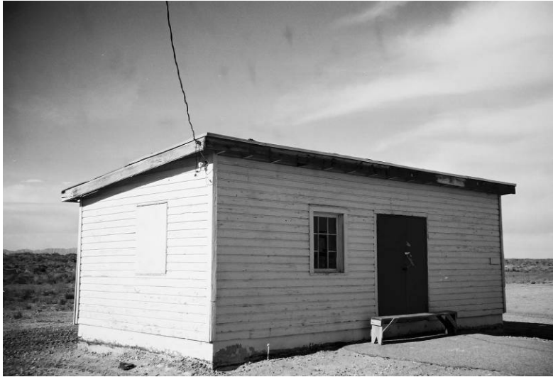
Figure 526. WWII Range Target Storage Bldg 9898, Fort Bliss, TX, November 2005.
