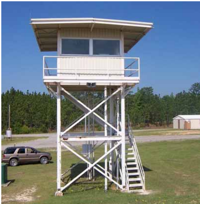
Figure 520. Observation tower, Fort Bragg, NC, 17 May 2006.
