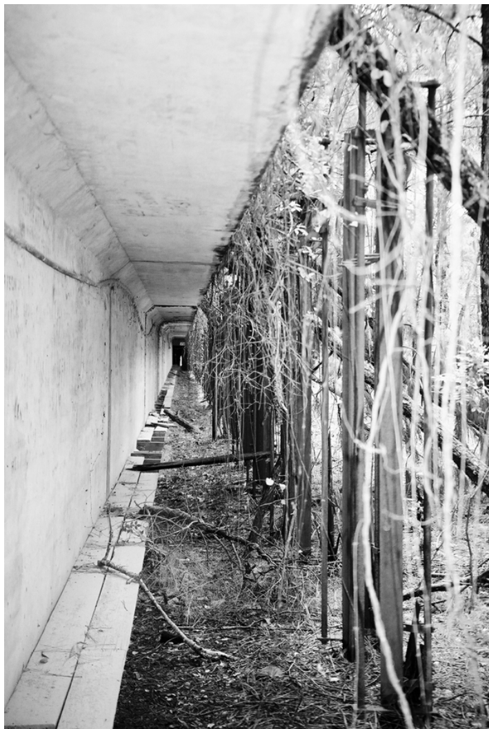
Figure 505. Remnants of WWII known distance range target butt, Fort Jackson (SCARNG), June 2004.
