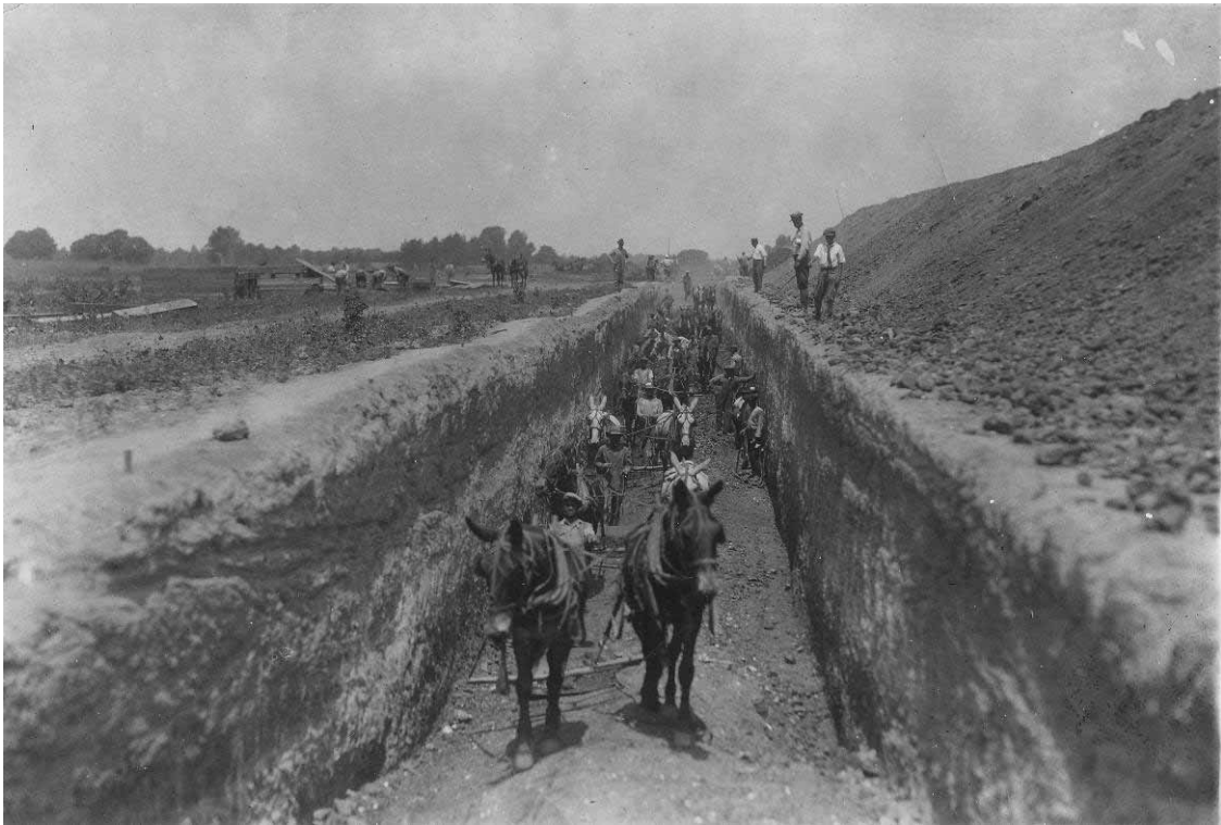
Figure 63. Horses digging target trench, Fort Knox, KY, undated (scans from Knox, training 6, vol. 5).
