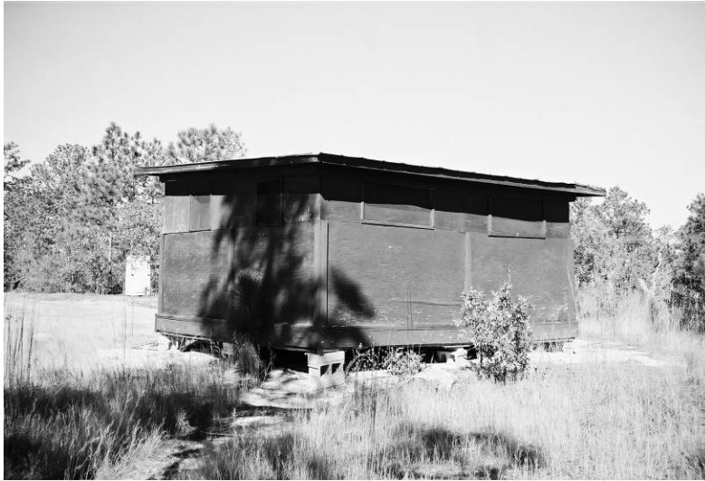
Figure 541. Remnants of WWII Latrine Bldg 9606, Fort Jackson, SC, November 2003.
