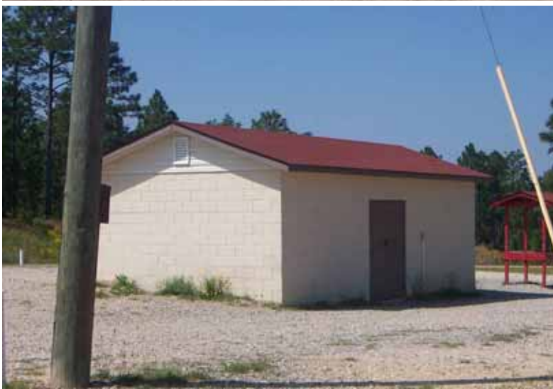
Figure 531. Range storage building, Fort Bragg, NC, 17 May 2006.
