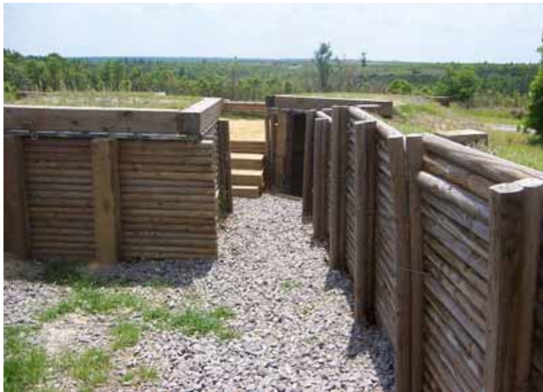
Figure 497. Walled embankments at grenade range firing lines, Fort Bragg, NC, 17 May 2006.
