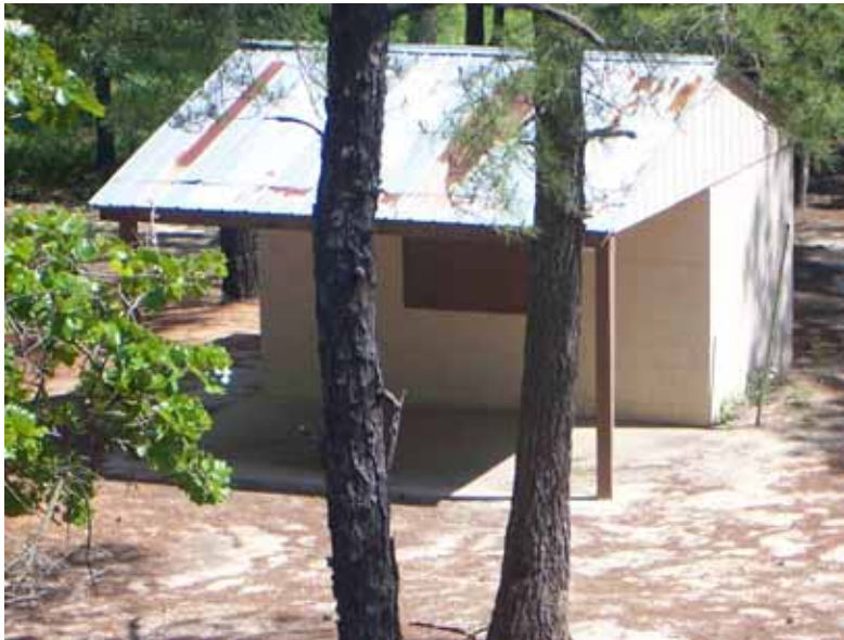
Figure 536. Range ammunition storage building, Fort Bragg, NC, 17 May 2006.
