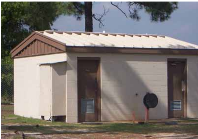
Figure 544. Range latrine, Fort Bragg, NC, 17 May 2006.
