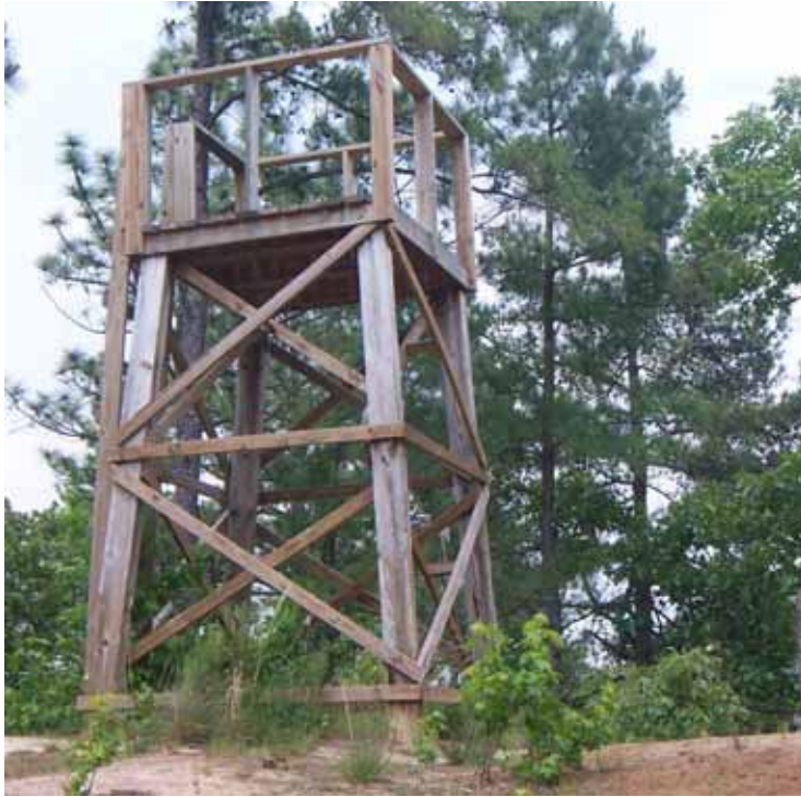
Figure 514. Observation tower, Fort Bragg, NC, 17 May 2006.
