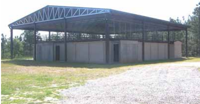
Figure 523. Range firing tower, Fort Bragg, NC, 17 May 2006.
