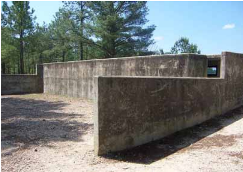
Figure 500. Grenade range protection walls, Fort Bragg, NC, 17 May 2006.
