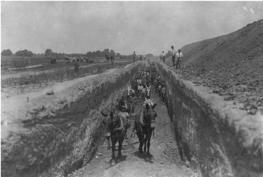
Figure 237. Horses digging target trench, Fort Knox, KY, undated (scans from Knox, training 6, vol. 5).
