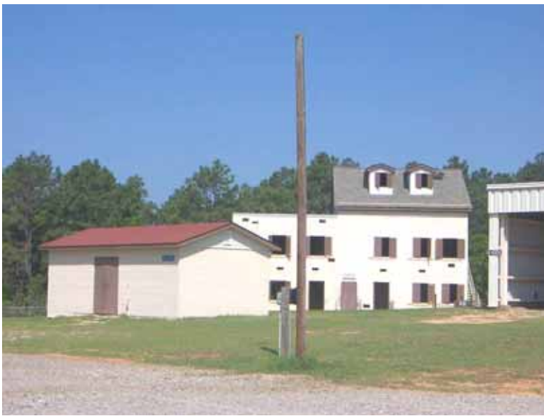
Figure 533. Range storage building, Fort Bragg, NC, 17 May 2006.
