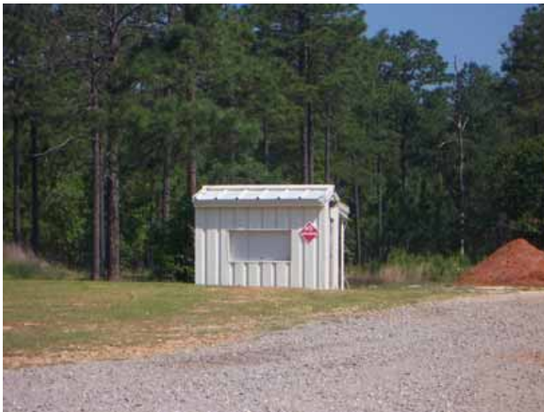
Figure 534. Range storage building, Fort Bragg, NC, 17 May 2006.
