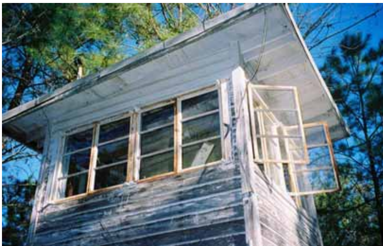
Figure 509. Remnants of WWII Observation Tower Building R122, Fort Gordon, GA, January 2004.
