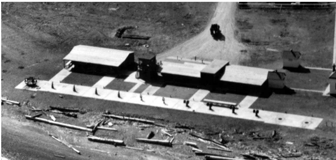
Figure 252. Machine gun range at Coast Guard Air Station Port Angeles, WA, 8 January 1957 (NARA College Park, RG 80-G, box 39, photo 7163).
