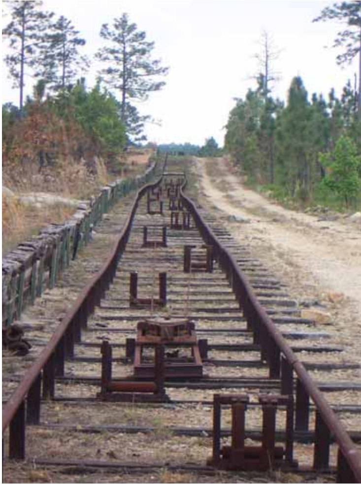
Figure 491. Cable pulley system on moving target track, Fort Bragg, NC, 17 May 2006.
