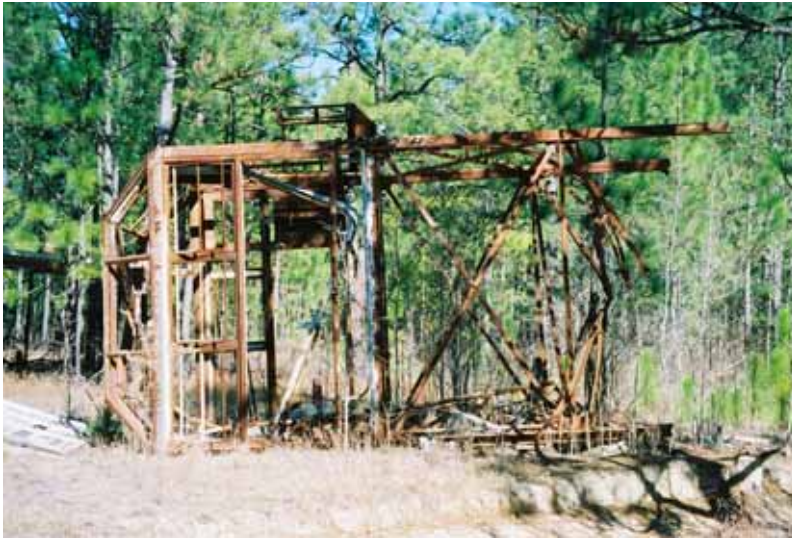
Figure 516. Remnants of 1966 Observation tower (near Building 421), Fort Gordon, GA, July 2004.
