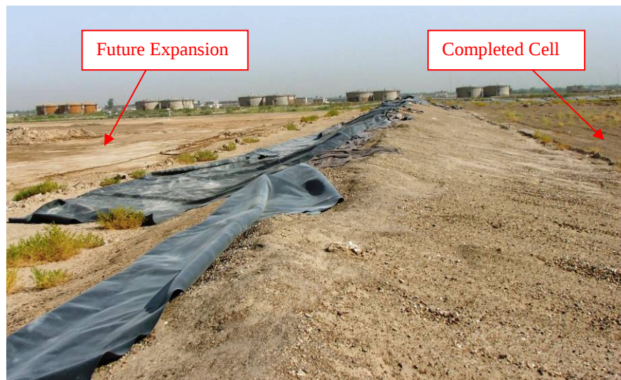
Site Photo 7. Interphase berm bordering future expansion area
