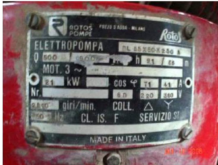
Site Photo 16. Factory plate for fire hydrant system pump (Photo provided by USACE)
