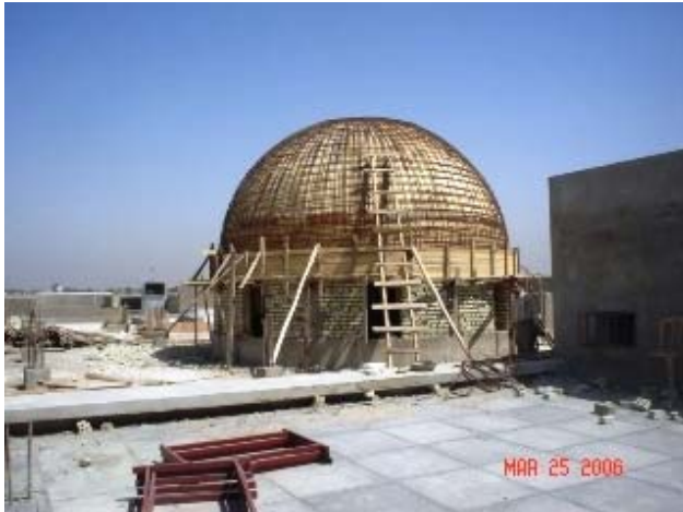
Site Photo 10. Dome after reinforcing steel installation (Photo provided by USACE)
