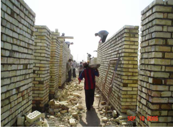
Site Photo 5. 36 cm walls on ground floor (Photo provided by USACE)
