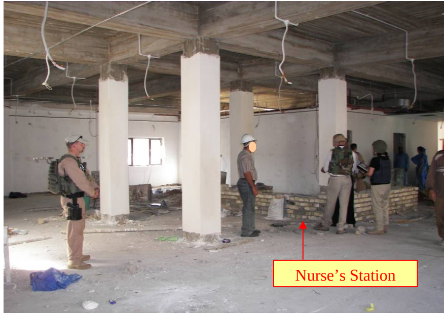
Site Photo 10. Ward area under construction.
