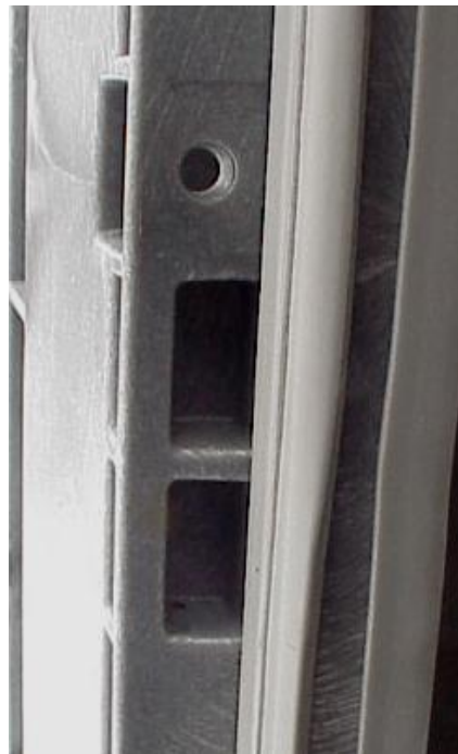
Figure 8. Blind openings for latch insertion; hole above for second lock.
