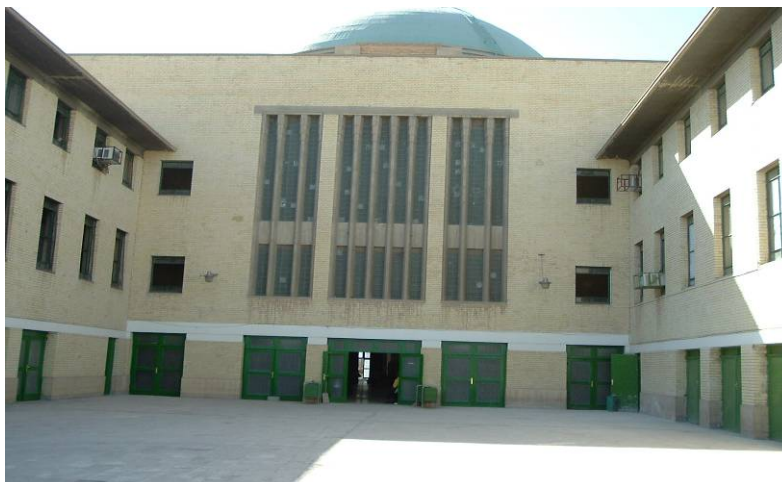
Site Photo 28. Rear view of railway station – site of future canopy
