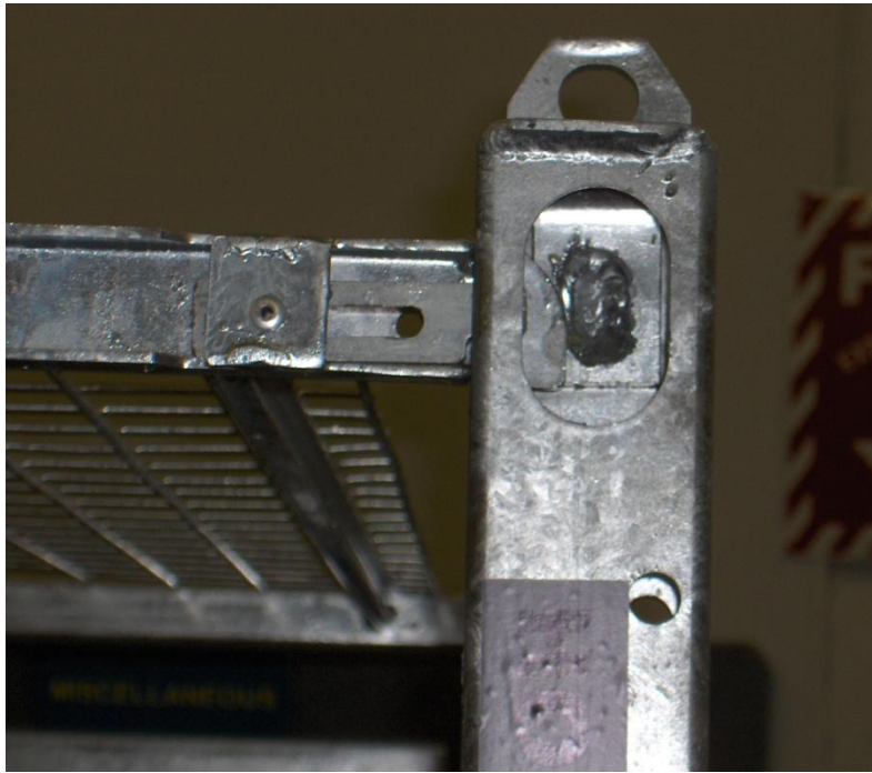
Figure 5. Corner post indexing tab and lockable slide for top panel.
