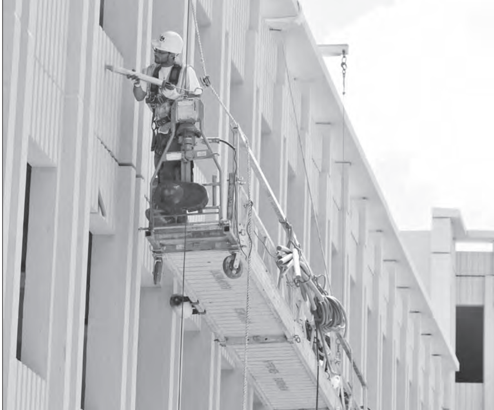
A contractor applies materials to seal the exterior wall of the south parking garage at the Department of Defense office complex (BRAC 133) project site.
