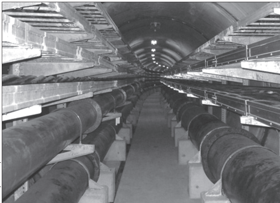
Medium-voltage cabling is supported by new cable trays in a Yokosuka Naval Base utility tunnel.
