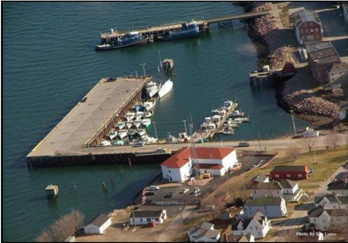
Figure 2: Eastport Breakwater and United States Coast Guard Station Eastport
