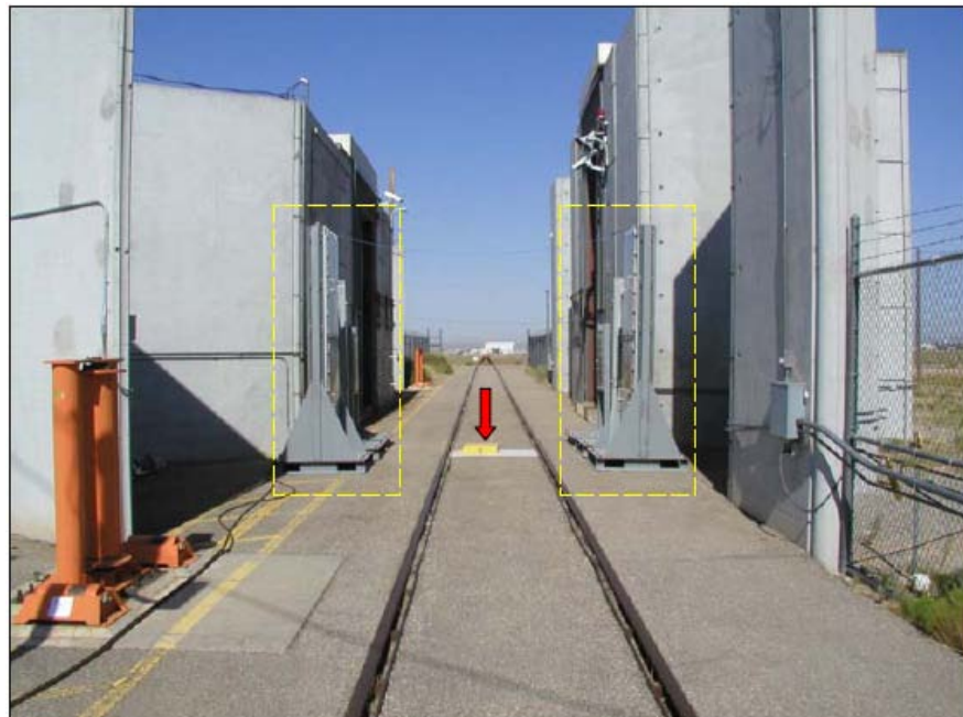
Figure 13. Picture of the DTRA TEAMS active neutron interrogation location at Kirtland AFB, NM (Grumman, 2004). The neutron generator is positioned in the hole below the red arrow.
