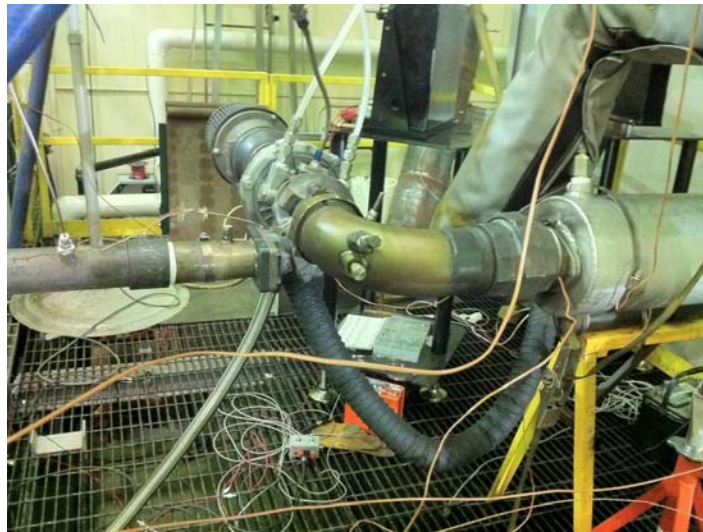
Figure III-15: Ten foot heat exchanger with turbocharger
