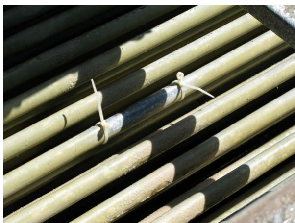
Figure 16. "After" photo of second clean section of upper tube of evaporative condenser at Zeta demonstration site (Davis Monthan AFB Fitness Center, September 2008).
