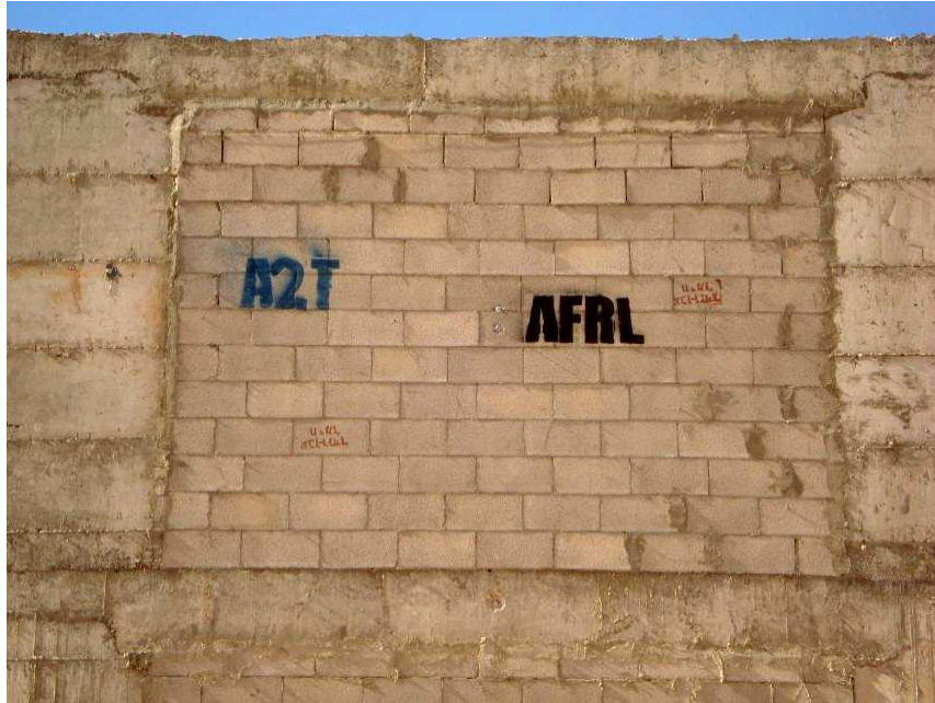
Figure 117. Pre-Test Photo (Exterior)
