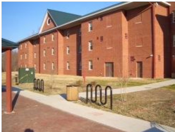
Figure 52 – Yorktown Bachelor Enlisted Quarters
