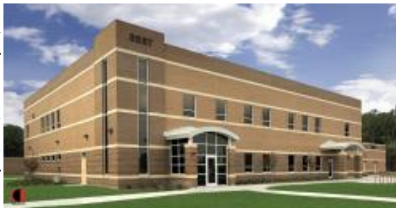
Figure 58 – Police and Security Operations Facility
