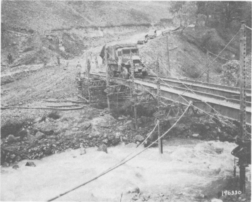
Figure 10. Short-gap fixed-bridge span.
