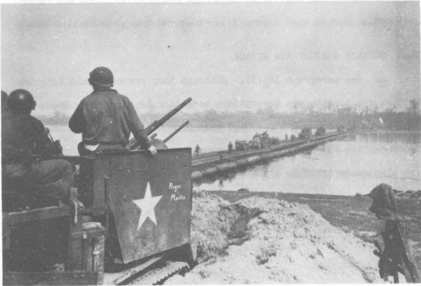
Figure 15. Antiaircraft guns emplaced to protect bridge against low-flying aircraft.
