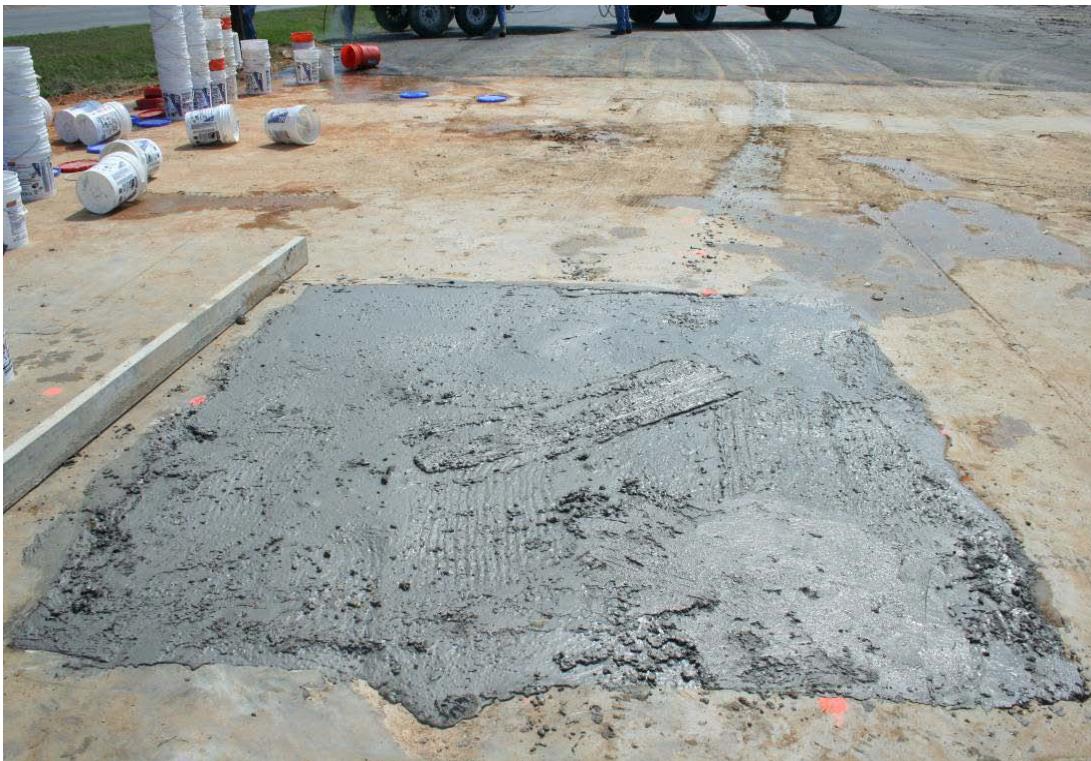
Figure 2. Pavemend TR surface.
