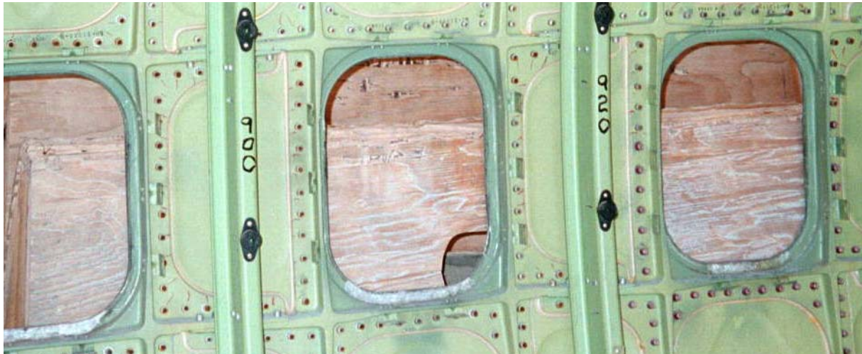
Figure 27-44: Lower Window Frame Corrosion Due to Moisture Accumulating Between Seal and Structure of Stored Airframe.
