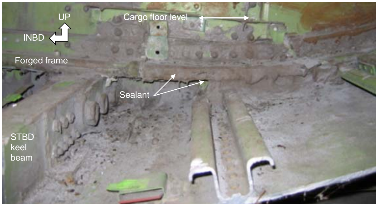
(b) View of area below cargo floor at fuselage frame, STBD.
