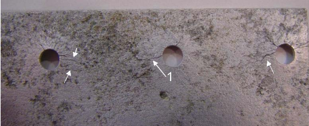
(a) Optical image of cracks in Boeing 707 longitudinal lap joints.
