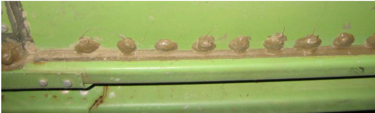
(a) Lap joint top row fasteners and stringer sealant application.
