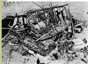
Wood Frame: 5 psi peak overpressure
