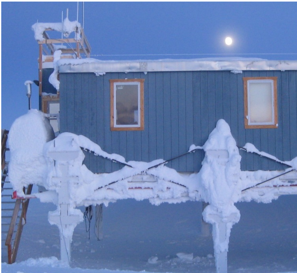
Figure 16. View 3 showing location (inset), thermal, and visual image of the eastern end of the North exterior wall in the vicinity of the office and main room.
