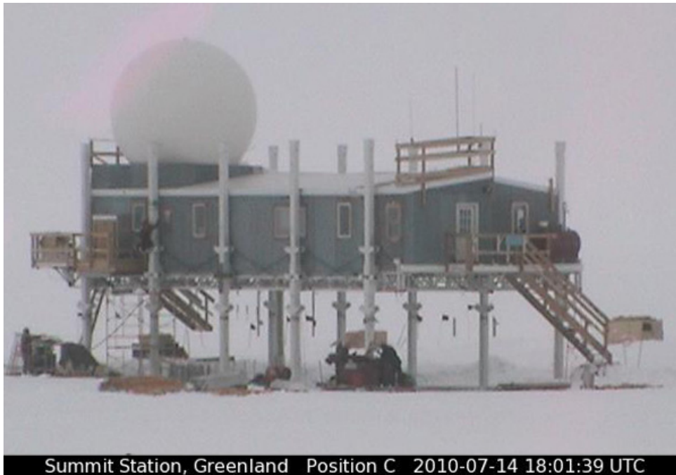
Figure 45. Completed lift of the Big House during the 2010 summer season.
