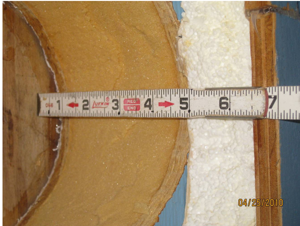
Figure 3. Big House wall material types and thicknesses.
