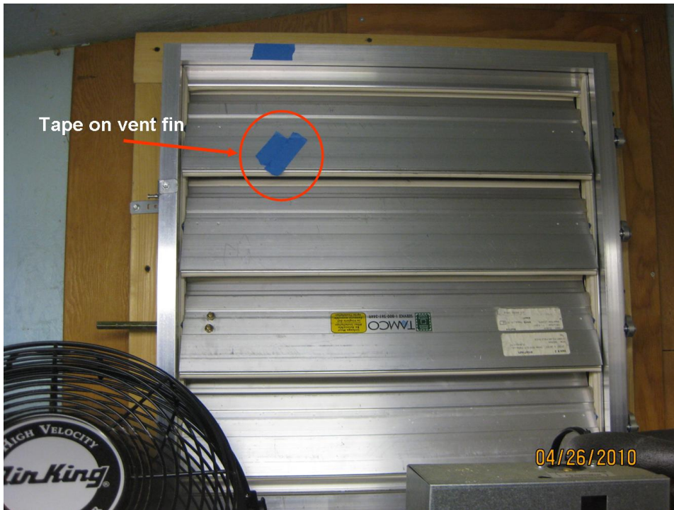
Figure 33. IR and visual imagery of the interior view of the large make up fresh air vent in the kitchen.
