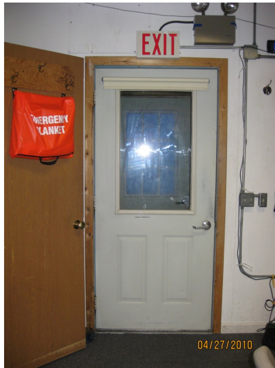
Figure 42. IR and visual images of the main entrance door in the east vestibule.
