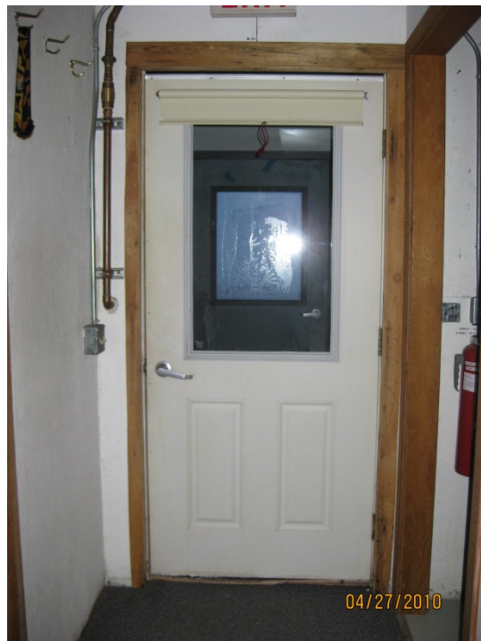
Figure 43. IR and visual images of the main entrance door in the west vestibule.
