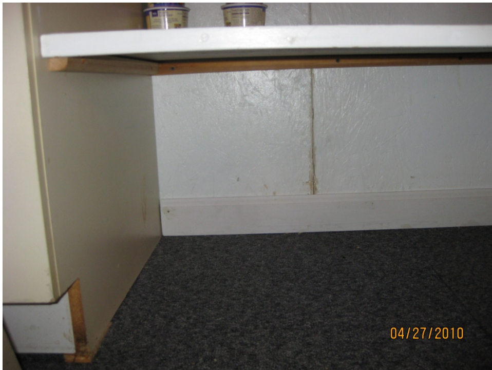
Figure 36. IR and visual images of the cold location under the counter in the main room before it was sealed.
