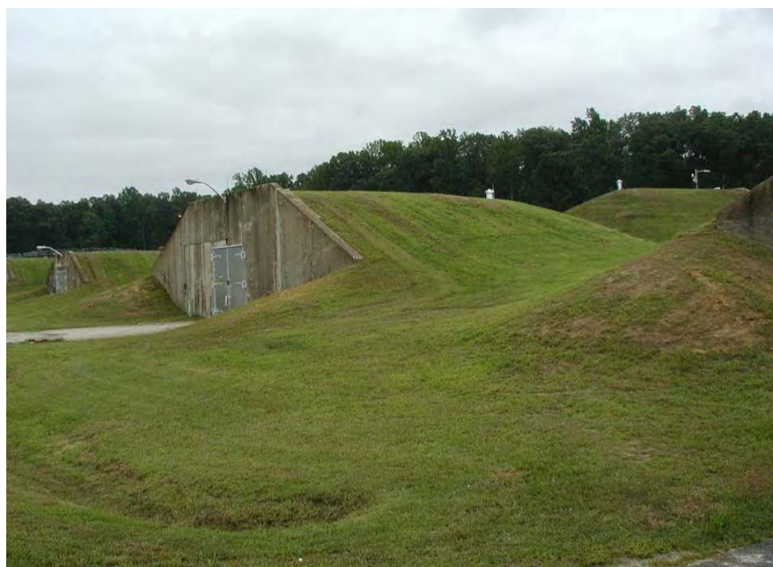
Figure 2.2. Typical steel arch earth-covered magazine.
