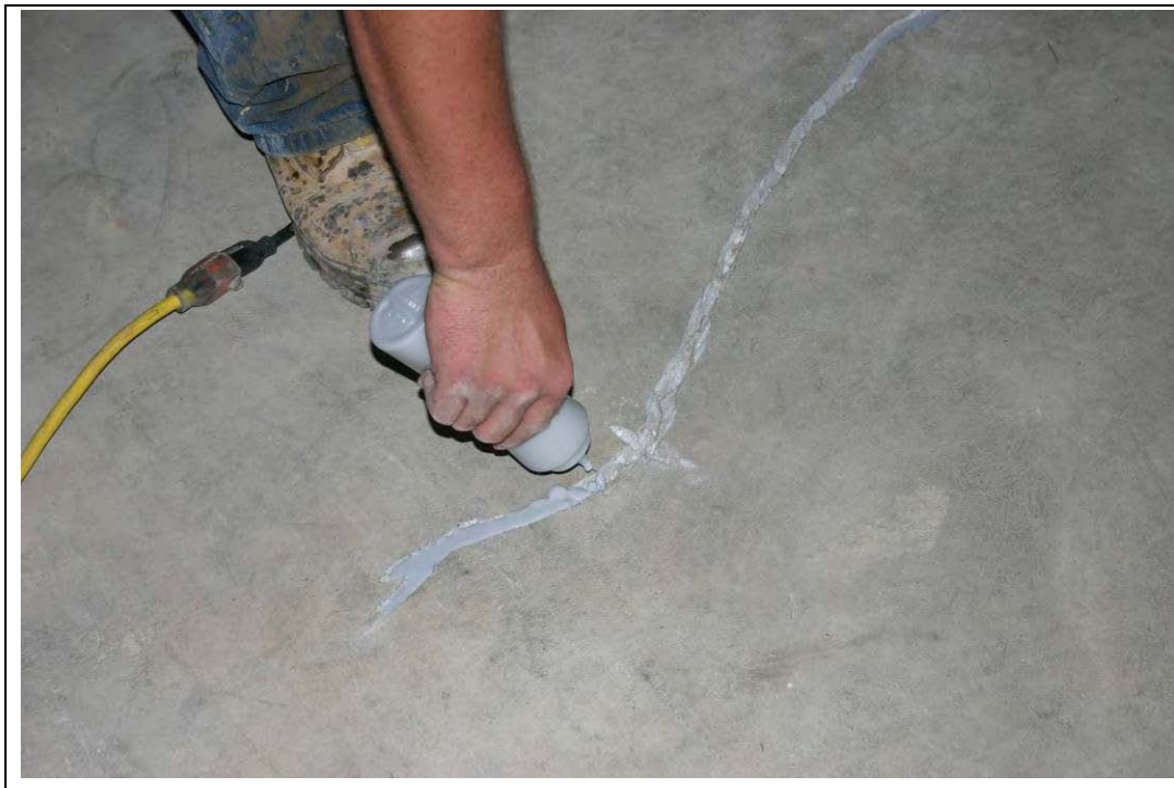
Figure E-8. Crack being filled with epoxy.
