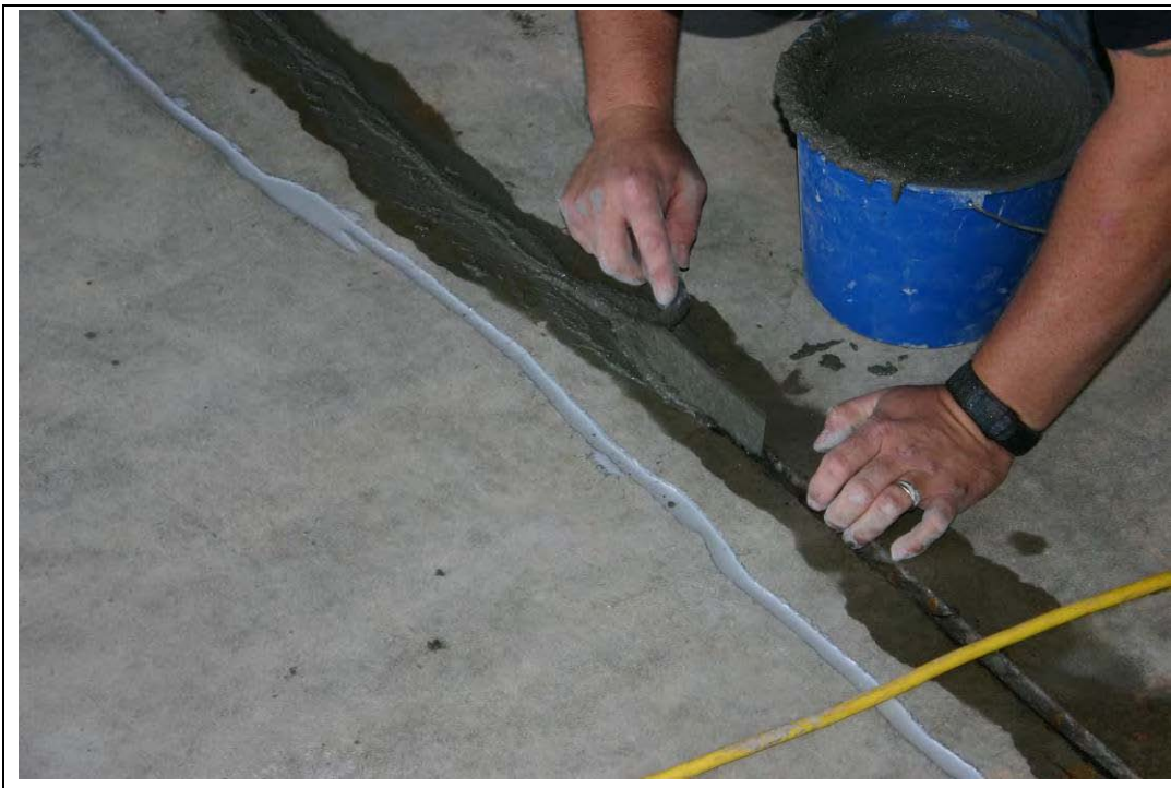
Figure E-18. Grouting of lead wires in prepared slot.
