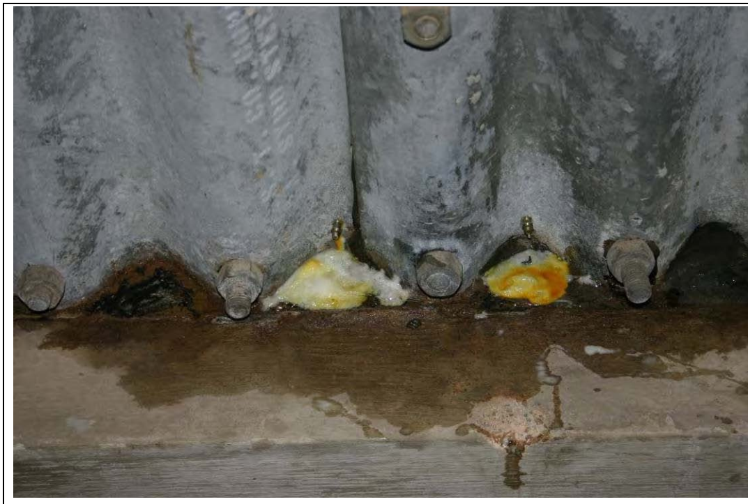
Figure E-27. Leak injection.
