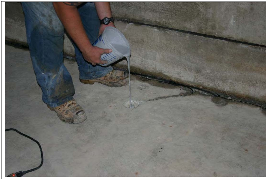
Figure E-14. Epoxy potting of cathode.
