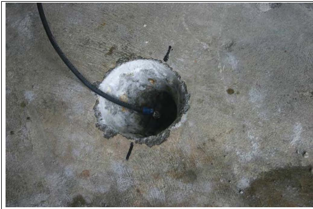
Figure E-16. Rebar lead wire connection.
