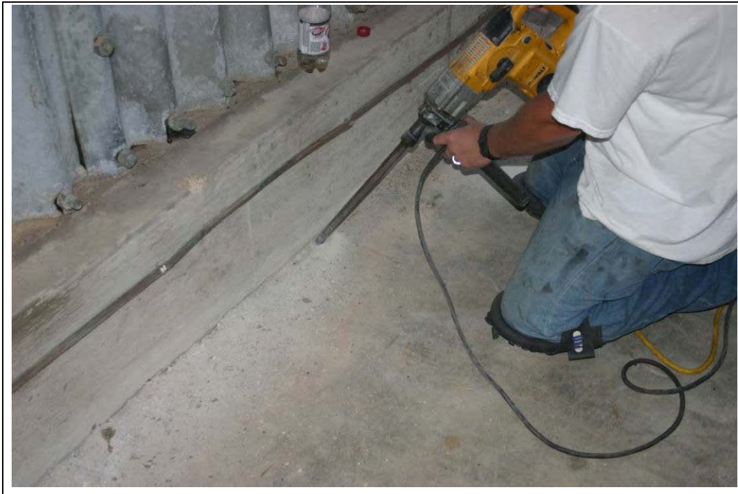
Figure E-3. Chipping of anode slot.
