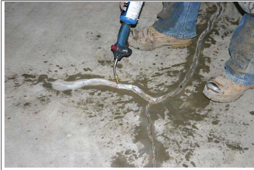
Figure E-7. Routed of floor cracks being dried following cleaning.
