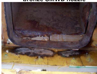
Galvanic Interaction at Bulkheads
