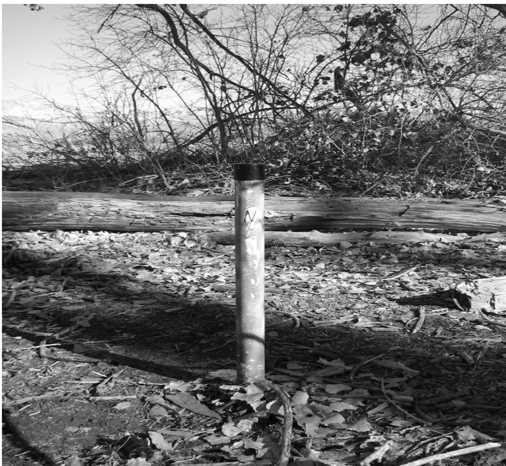
Figure 3. Typical well casing above ground.
