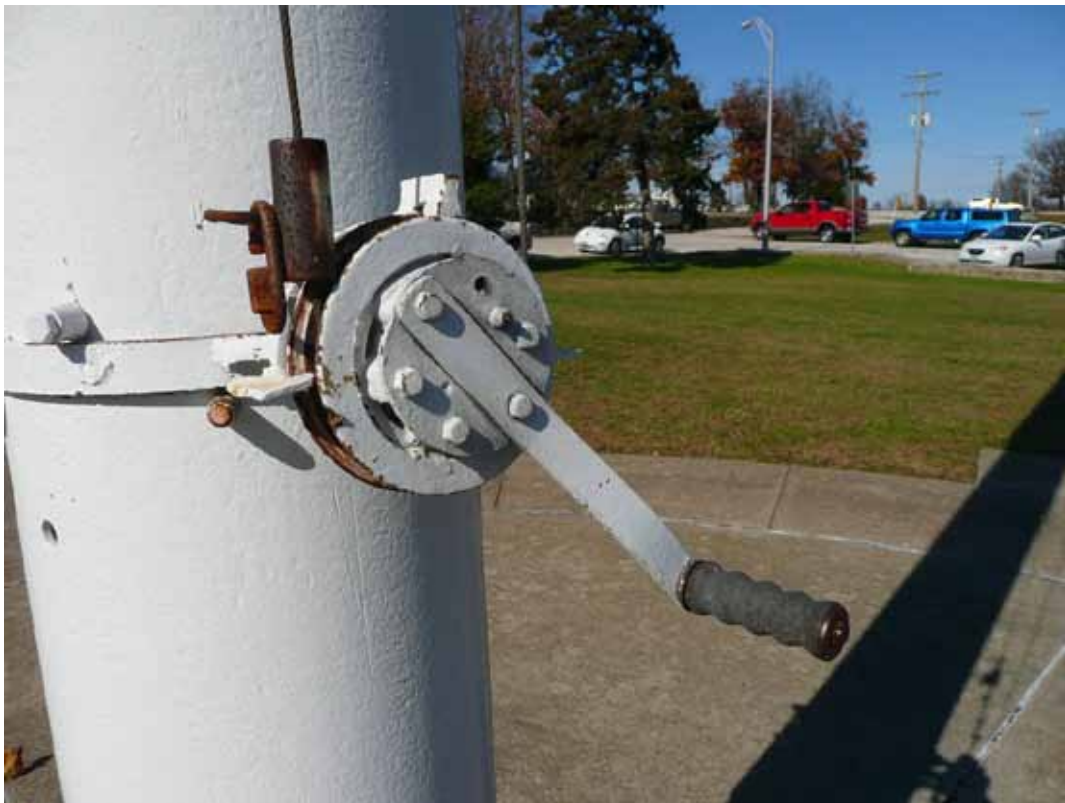
Figure 37. Detail of flagpole hand crank.
