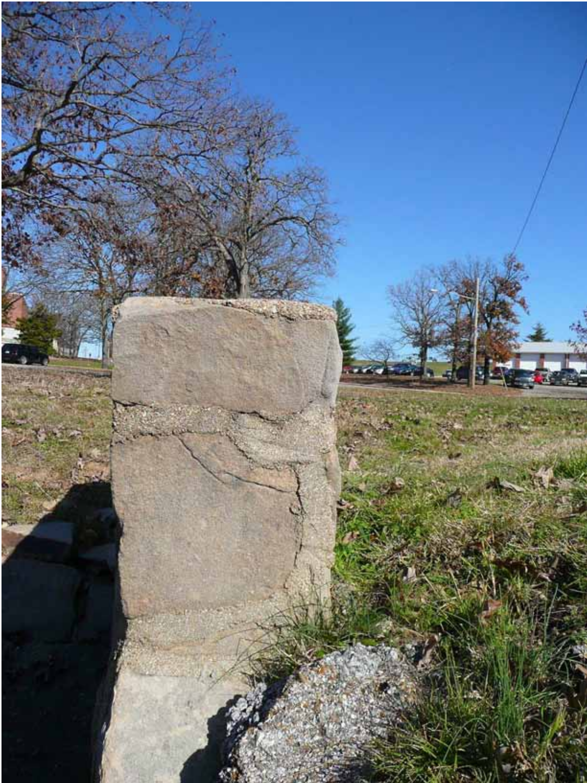
Figure 17. South elevation, west end of culvert.
