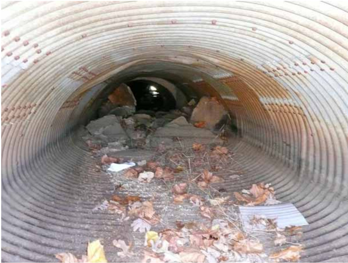
Figure 20. Inside west end of culvert.
