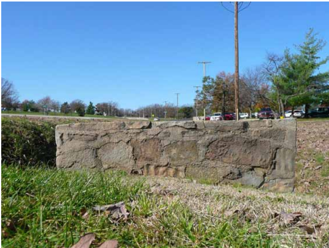
Figure 15. East elevation, west end of culvert.
