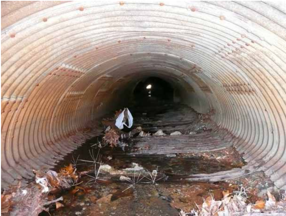
Figure 7. Inside of culvert, east end.
