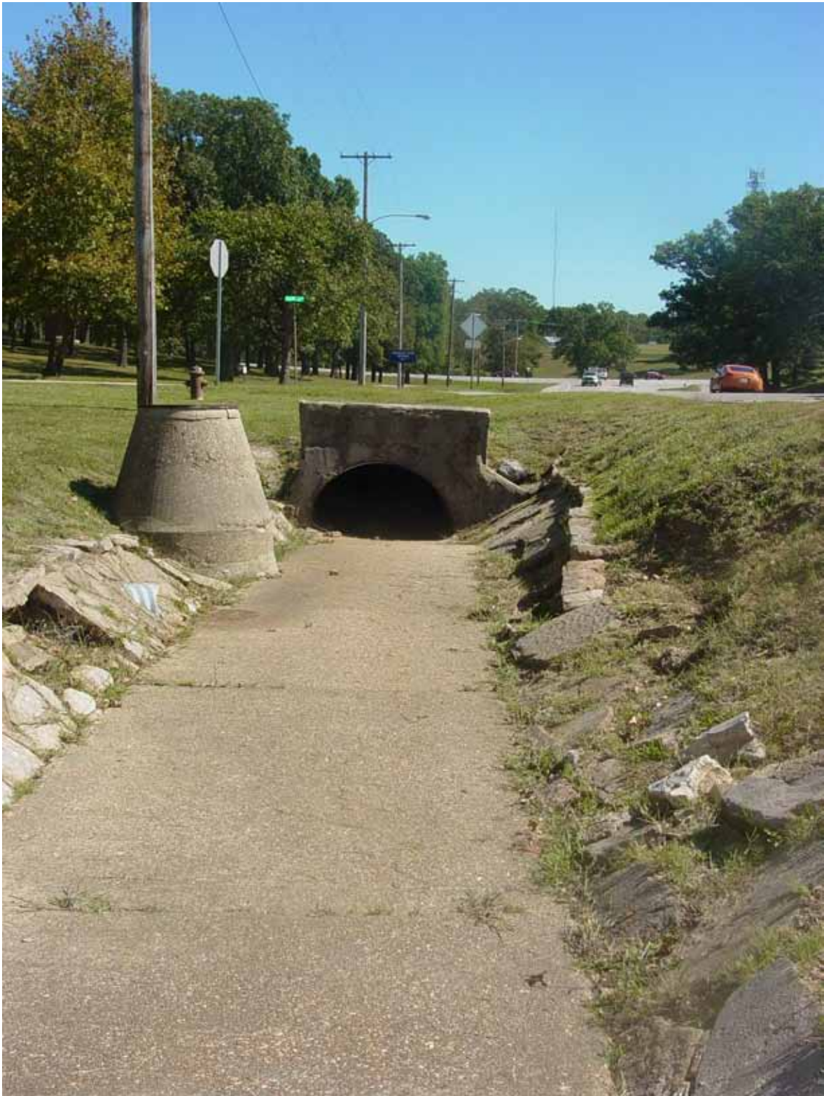
Figure 26. Overall elevation, west end of culvert.
