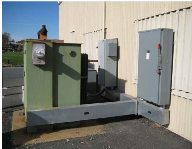
Figure 14. Warehouse Buildings – metal cladding.
