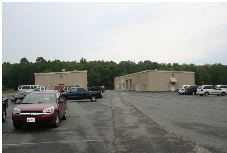
Figure 12. Warehouse Buildings – side view.
