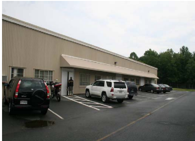
Figure 13. Warehouse Buildings – entry.
