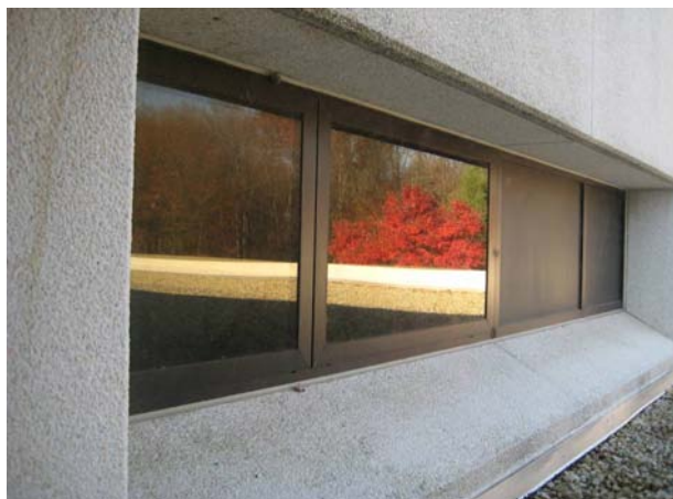
Figure 10. Casey Building windows.
