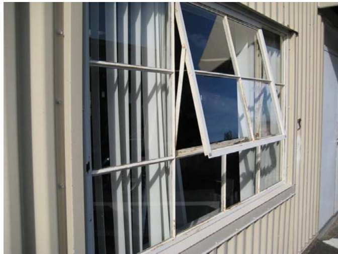
Figure 15. Warehouse Buildings – windows.
