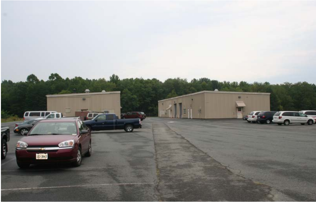
Figure 19. Fitness Center/Mailroom and Museum/Motor Pool Buildings
