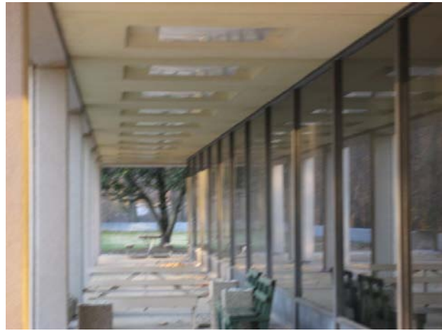
Figure 4. Kingman Building curtain wall.
