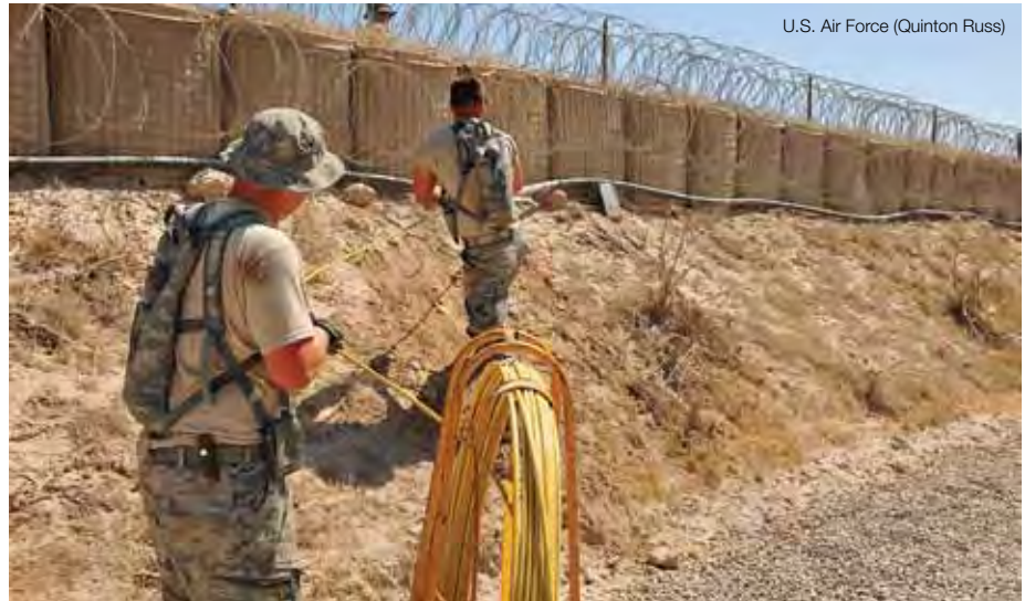
Airmen prepare to run fiber optic cables to improve connectivity at Camp Herat, Afghanistan
