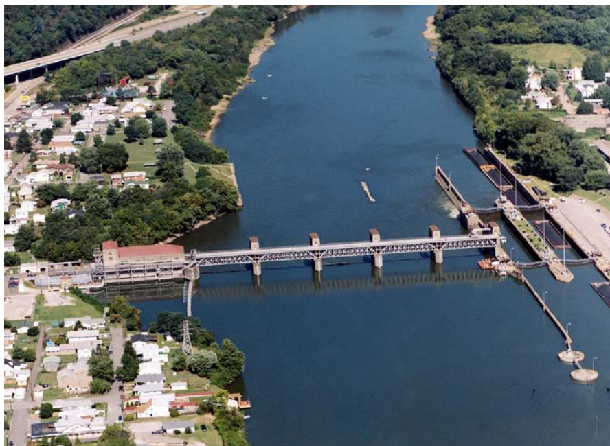
Figure 5.17 Marmet Lock and Dam with Cellular Bullnose
