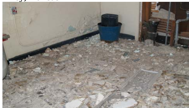
Figure 2. Interior of Building 216 at Fort Riley, Kansas
