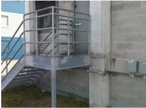
Photo 4: Exterior view of training tower doorway
