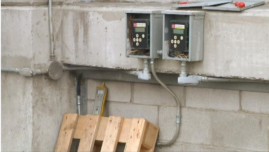
Photo 3: Installed thermocouple System and improvised set-up.
