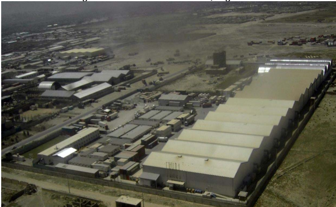
Figure 1. PV's Warehouse–Kabul, Afghanistan
