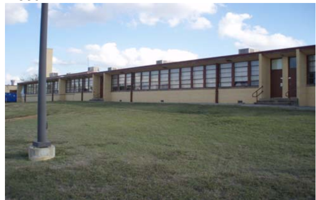
Figure 2. Exterior of Building 422 at Fort Hood
