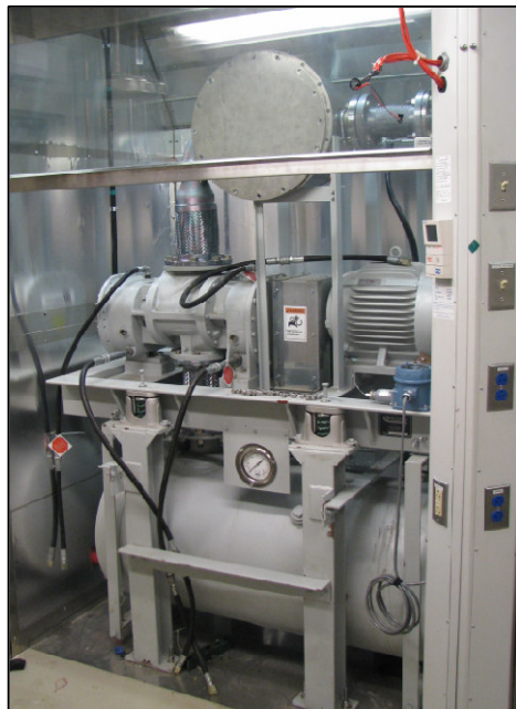
Figure 12. CBART Blower Assembly Installed in the 6-ft Hood
