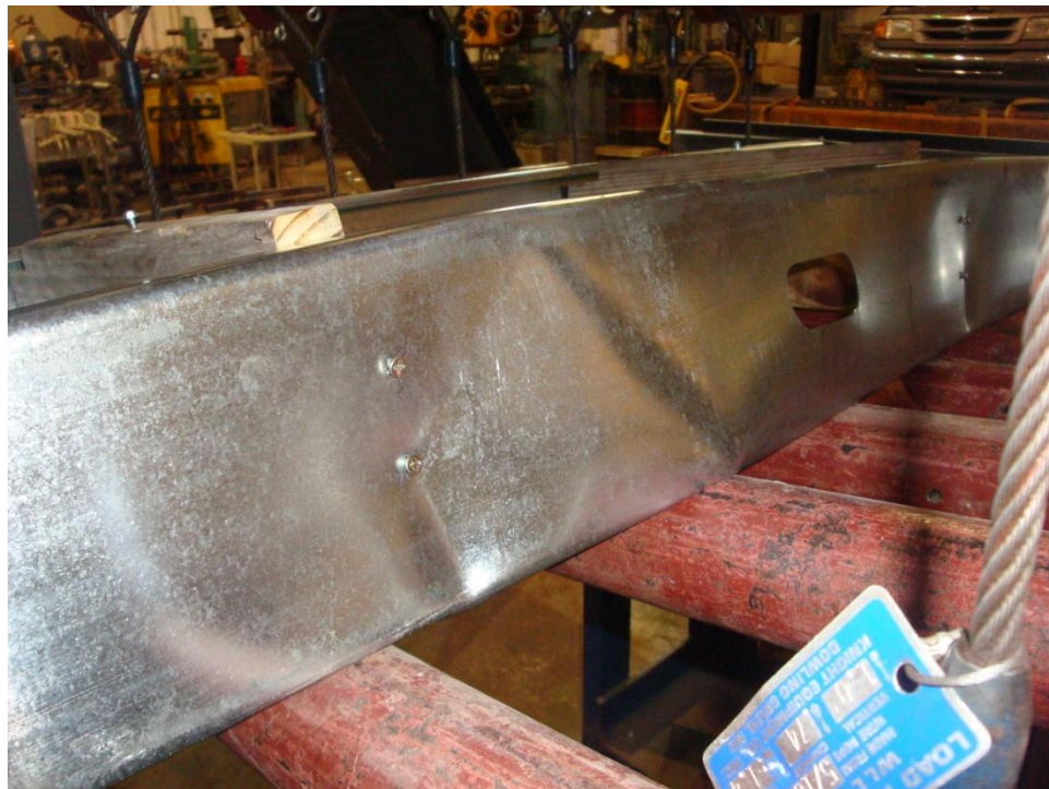
Figure B-32. Full-Length Sample 51 after Failure
