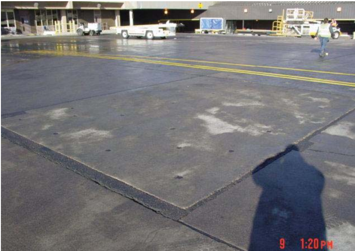
Figure 9. Precast Slab Replacement at the Calgary International Airport [27]
