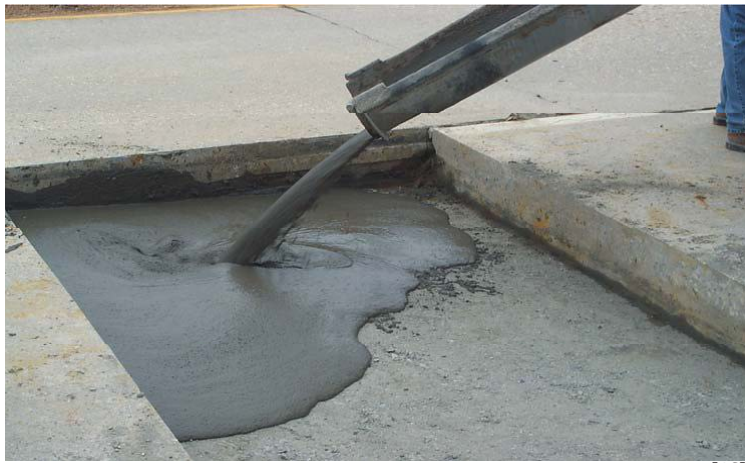
Figure 12. Flowable Fill Used by Michigan Method [16]
