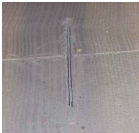
Figure 8. Fiberglass Ties Installed in a Transverse Joint [9]
