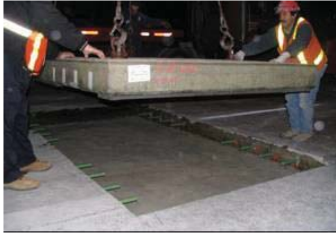
Figure 4. Installation of a Single Precast Panel on a Highway Using Fort Miller Method [17]
