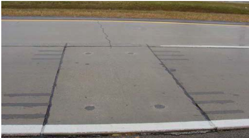
Figure 18. Completed Repair Using Michigan Method [16]
