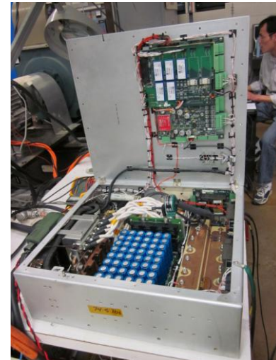
Figure 6 Vehicle Power Converter (VPC)
