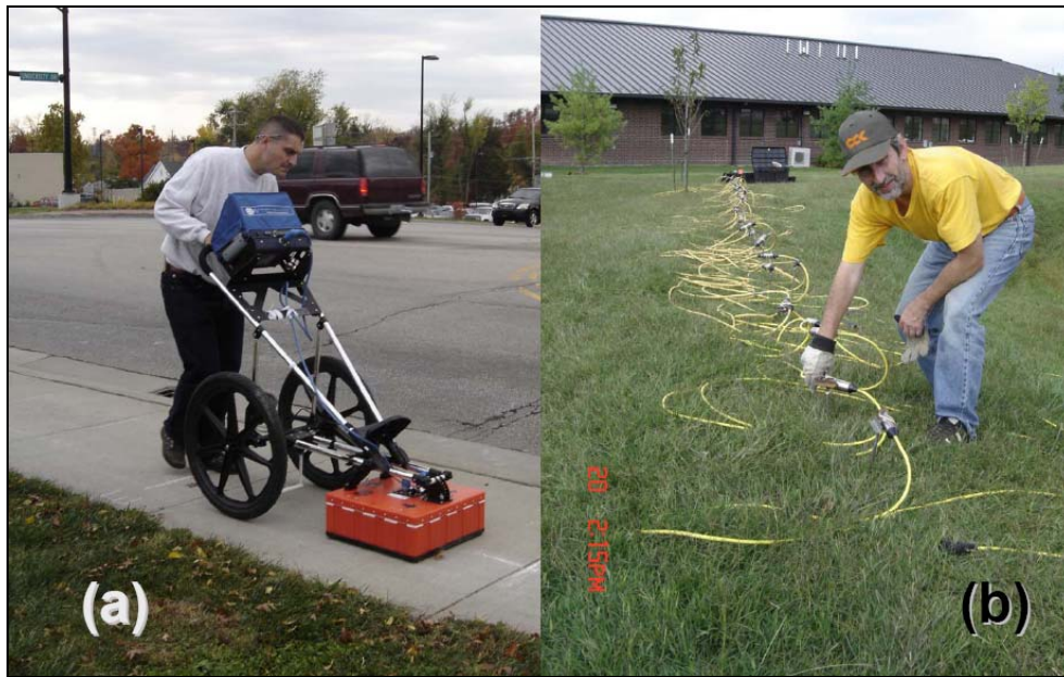
Figure 6.1: Missouri S&T Graduate Students conducting geophysical tests; (a) GPR with a 400 Hz antenna was used on asphalt and concrete, and (b) electrical resistivity was used for soil as the respective complementary geophysical methods.
